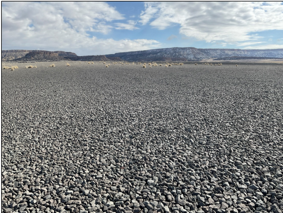
PL-6. Vegetation on Disposal Cell Top Slope
