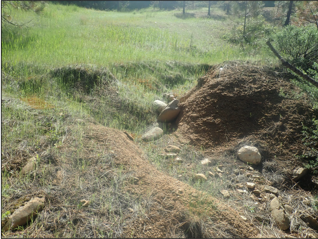
PL-7. Erosion on North Side of Interceptor Benches
