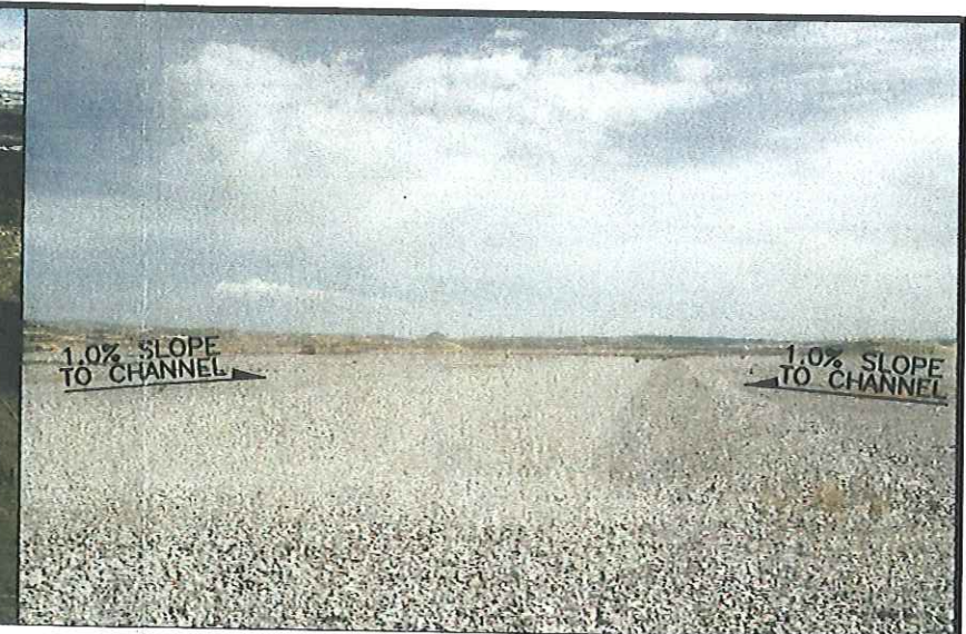
CHANNEL ON TOP OF HEAP LEACH REPOSITORY
