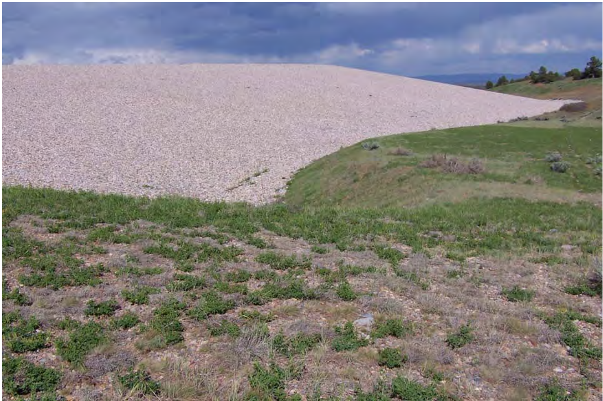
DUR 5/2008. PL-3. South side slope of cell; note absence of woody vegetation.
