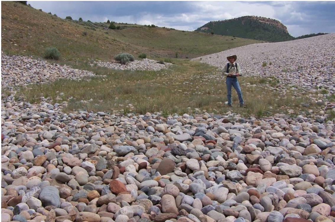
DUR 6/2006. PL-2. Sediment deposition in Diversion Channel No. 1.
