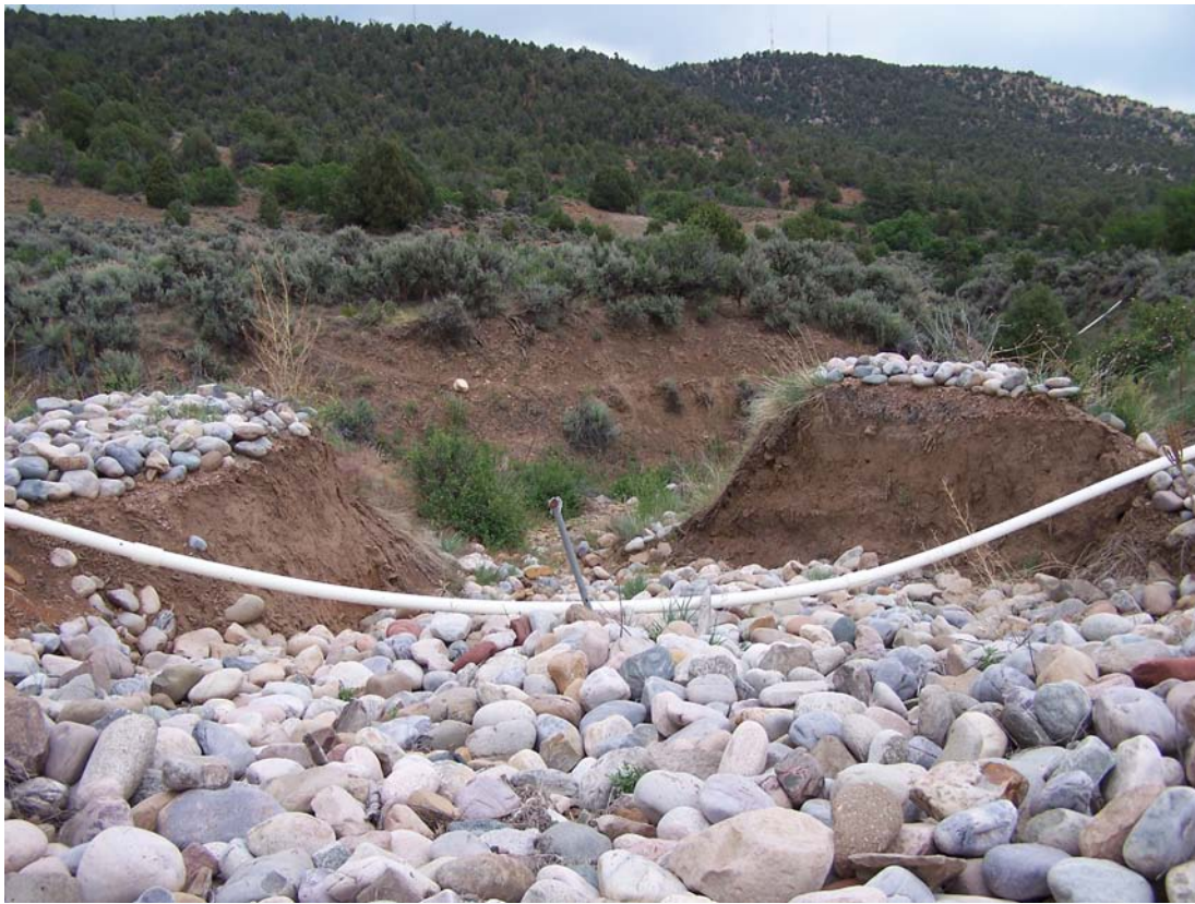
DUR 6/2006. PL-3. Northeast Outflow; no new erosion.
