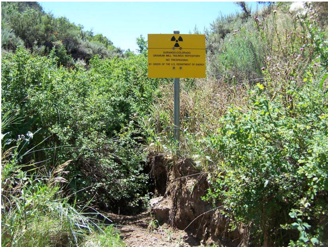
DUR 8/07. PL-2. Undercutting and deposition at perimeter sign P44.
