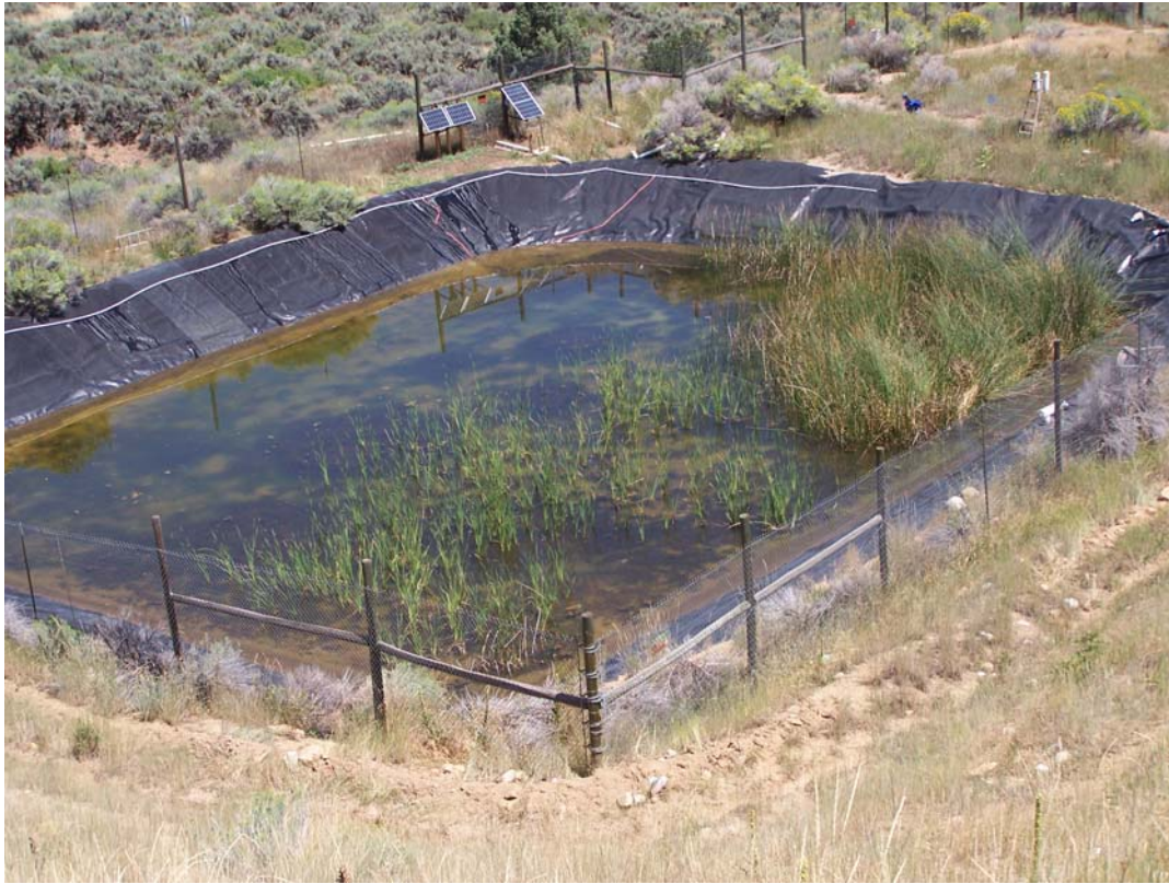
DUR 8/07. PL-5. Retention pond; note drip lines along top and left banks.
