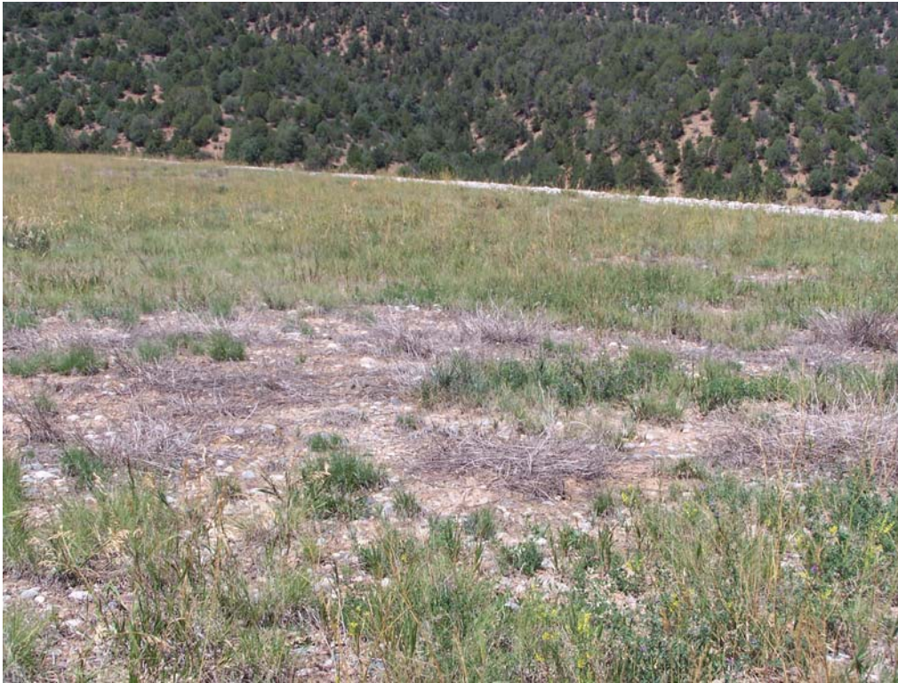
DUR 8/07. PL-3. Dead alfalfa plants on disposal cell top, sprayed with herbicide in September 2006.
