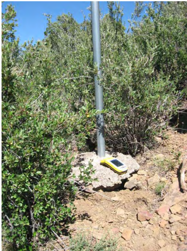
DUR 6/2010. PL-1. Undercutting at perimeter sign P41.
