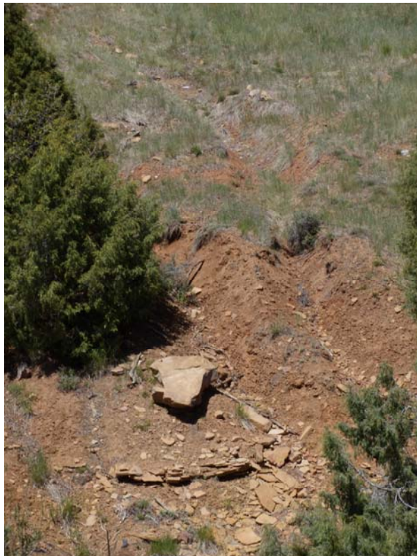
DUR 5/2011. PL-4. Headcuts of gullies below southwest corner of disposal cell; no change from 2009.
