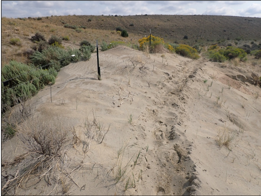
PL-15. Sand Accumulation Along Southern Fence Line Near Johnson Pit
