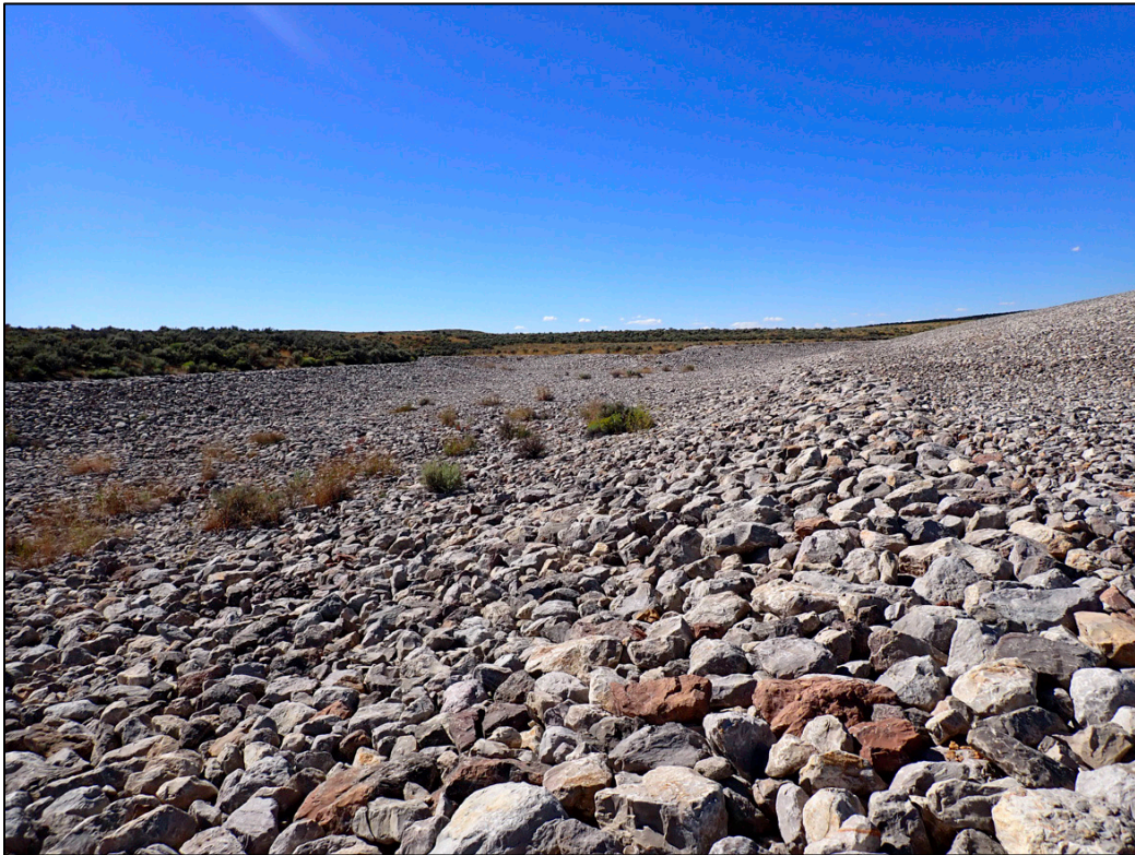
PL-5. Diversion Channel No. 1
