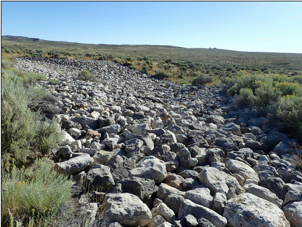
PL-6. Gully No. 4 Overview
