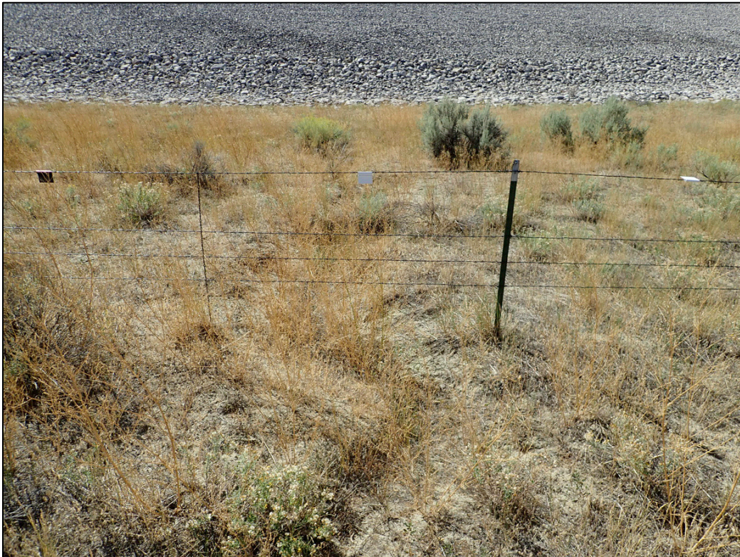
PL-10. Minor Rilling Under Fence
