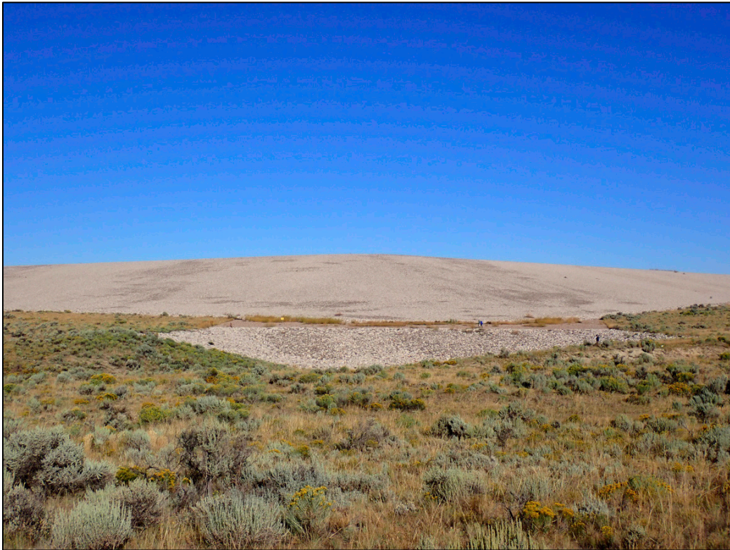
PL-3. Disposal Cell Overview
