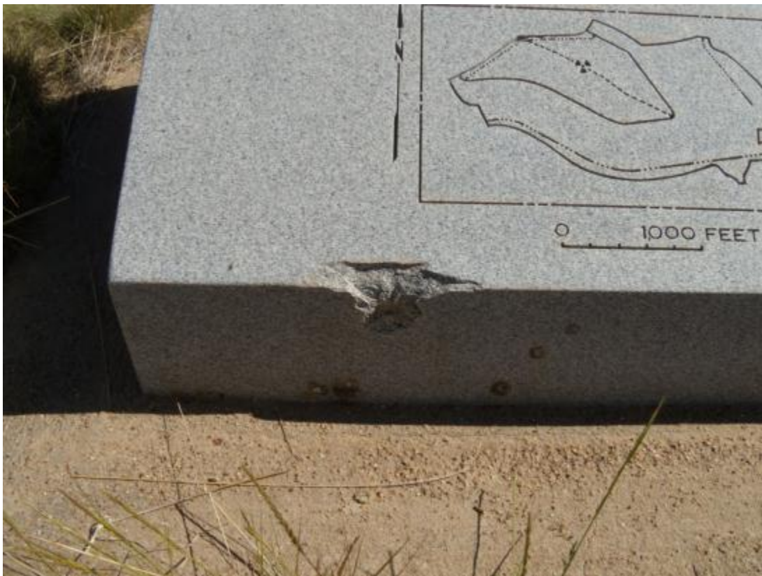
DUD 5/2012. PL-2. Chipped portion of site marker SMK-1.
