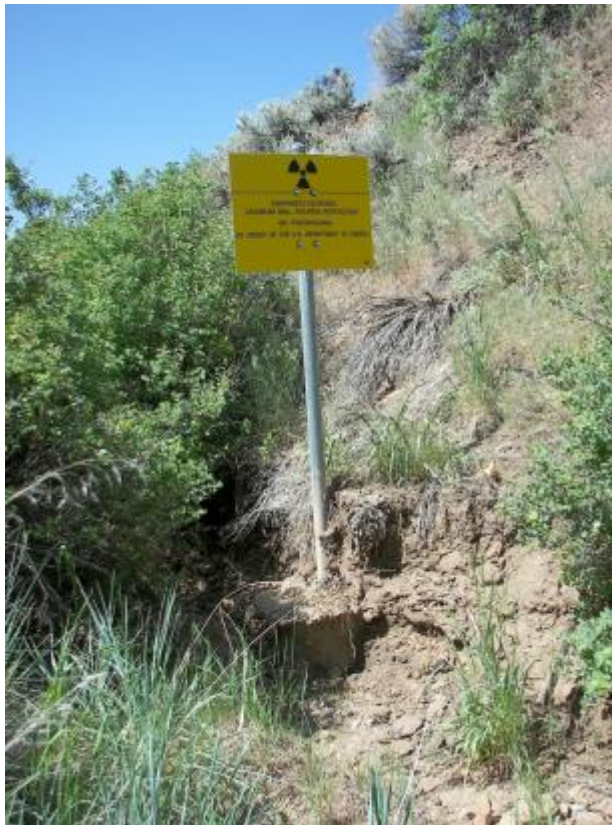
DUD 5/2011. PL- 1. Perimeter sign P45, showing undercut area.
