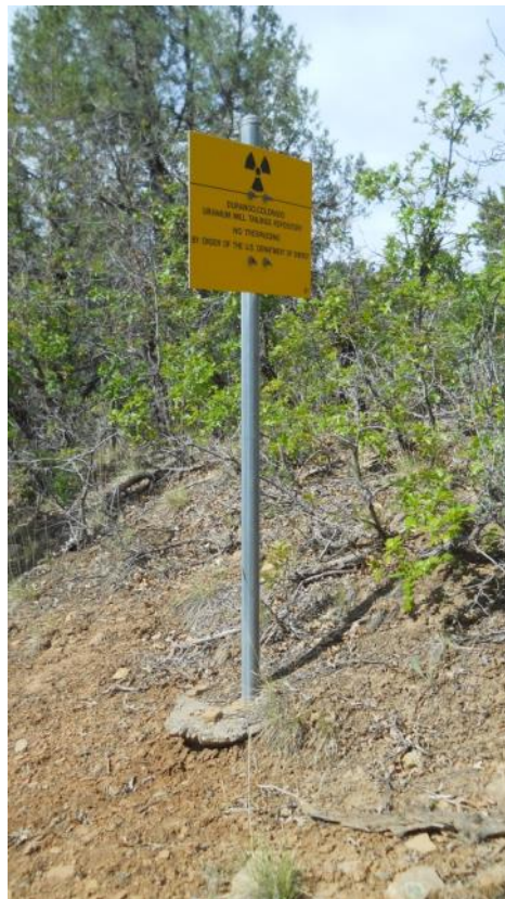
DUD 6/2014. PL-2. Perimeter sign P61 showing minor undercutting.
