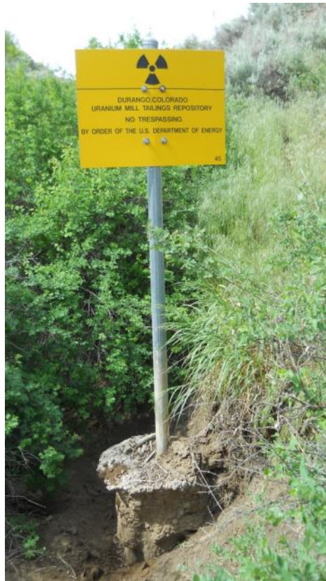
DUD 6/2014. PL-1. Perimeter sign P45 with significant undercutting.
