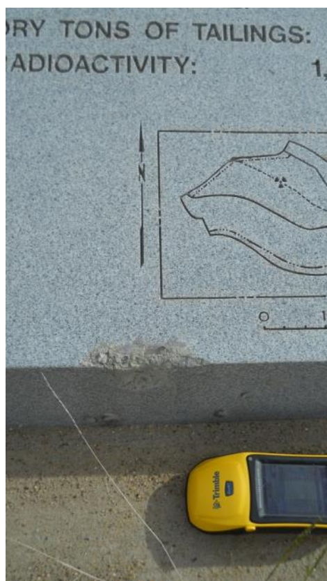
DUD 6/2014. PL-3. Site marker SMK-1 in need of repair.
