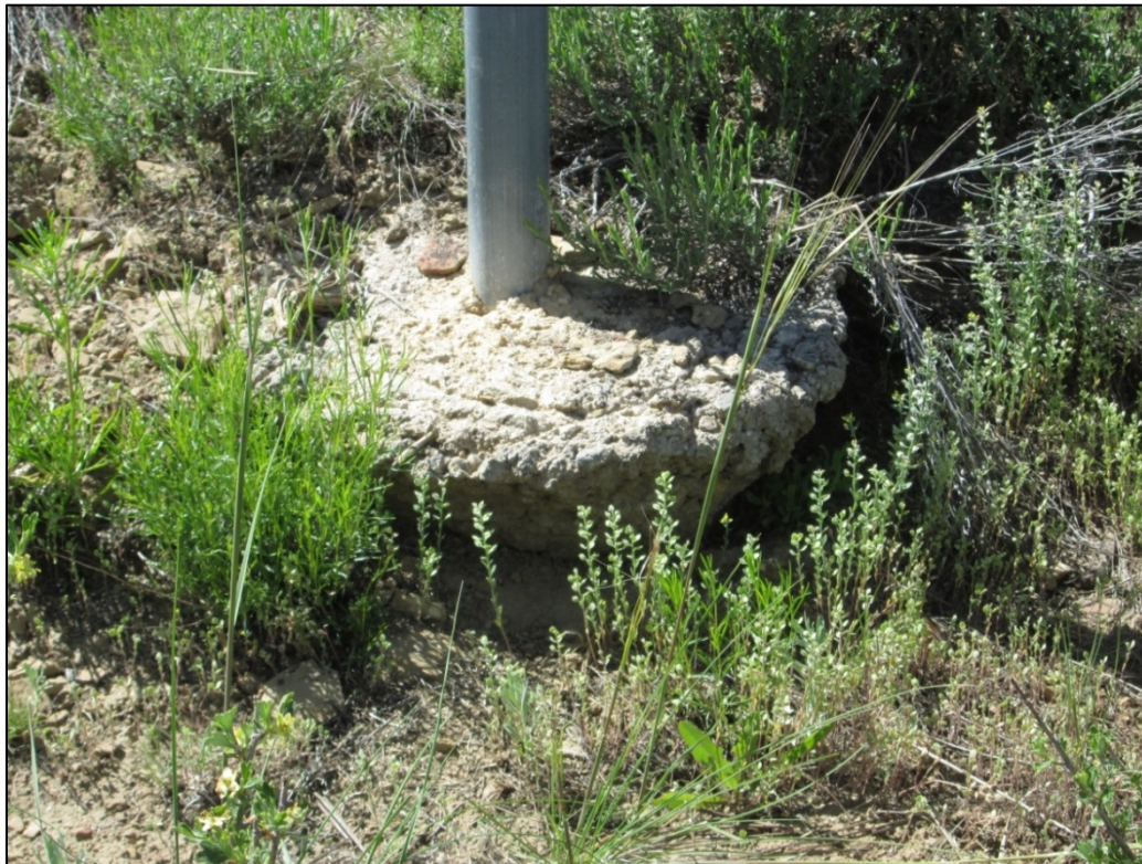
PL-2. Base of Perimeter Sign P38, With 3–4 Inches of Erosion on Downslope Side
