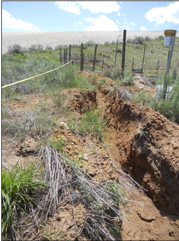
PL-11. Ditch Installed Around Evaporation Pond to Reduce Inflow Before Pond Removal
