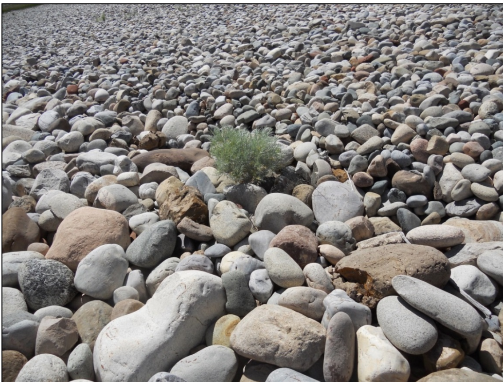
PL-8. Area of Disposal Cell Toe Where Rock Movement Has Occurred, 2015
