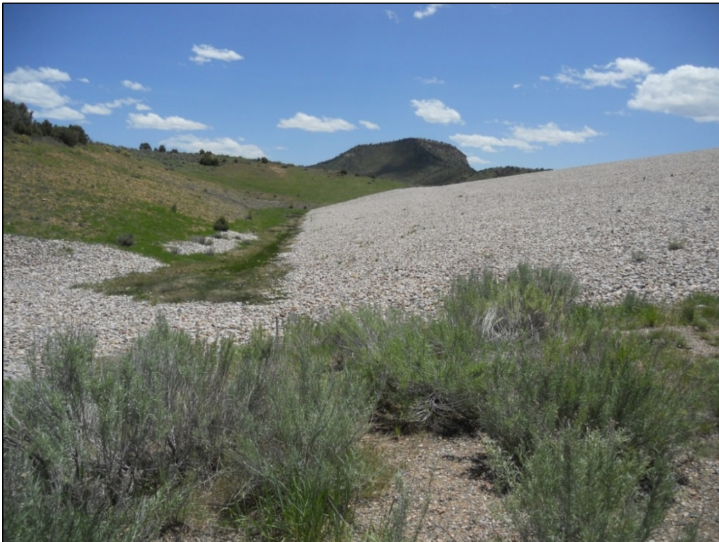
PL-10. Ditch No. 1 Showing Sediment Deposition and Vegetation Growth
