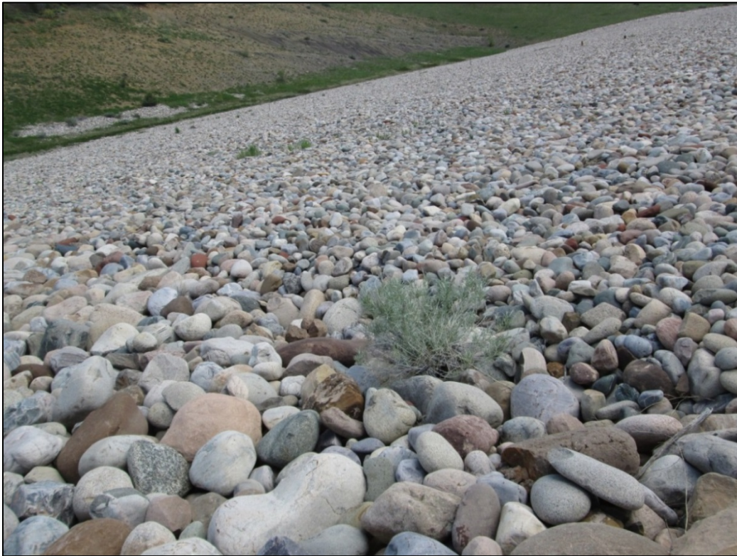
PL-9. Area of Disposal Cell Toe Where Rock Movement Has Occurred, 2016
