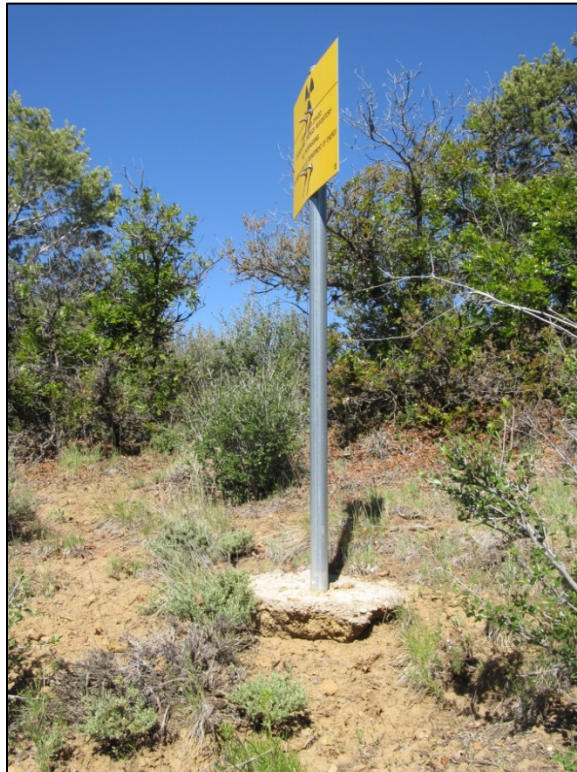
PL-3. Perimeter Sign P13, Undercut by Erosion
