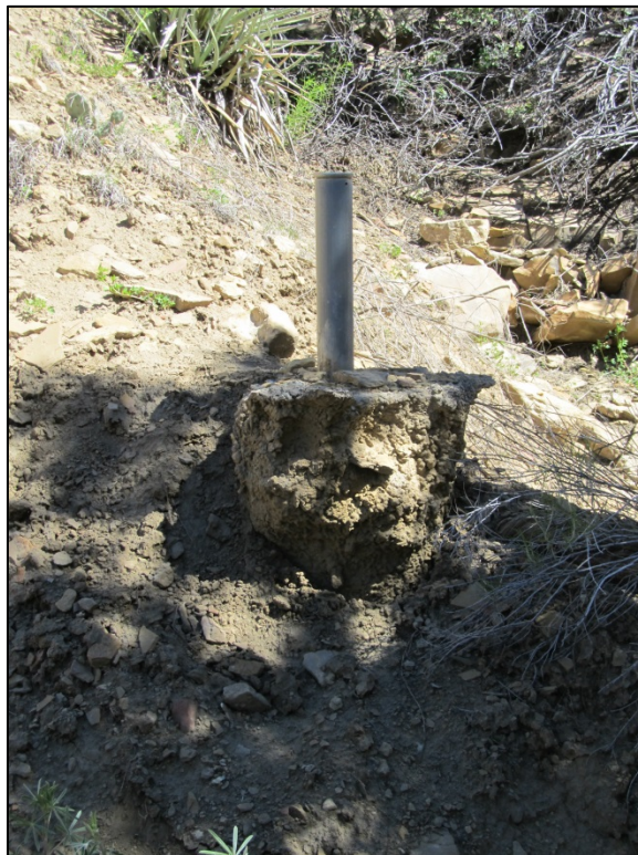
PL-6. North Reference Marker at Boundary Monument BM-3, Erosion at Base; Needs Stabilization
