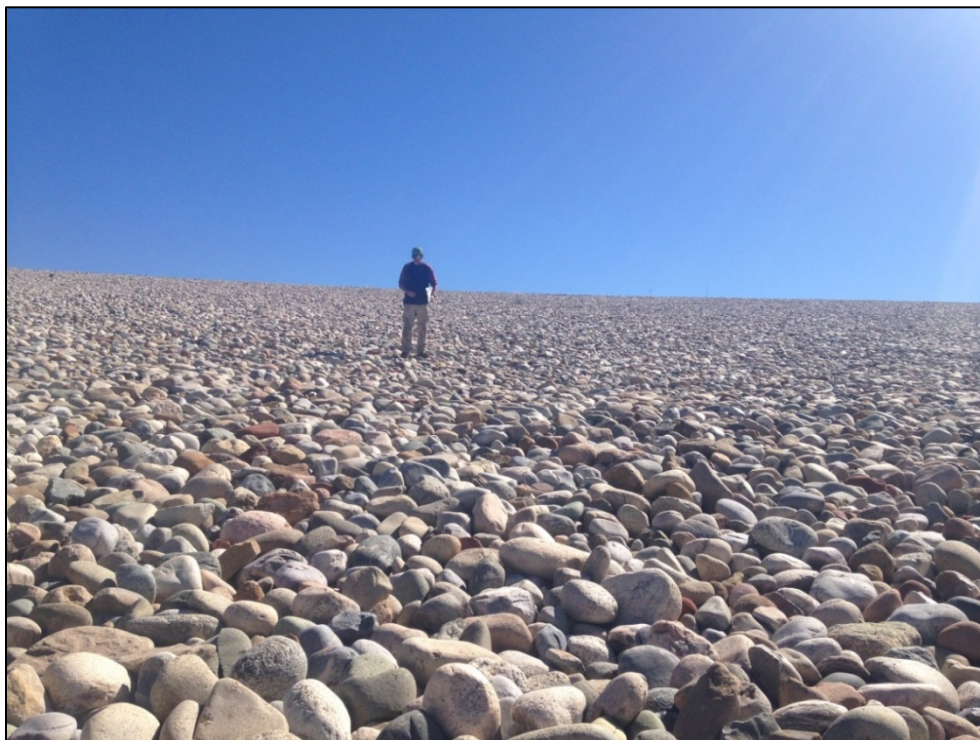
PL-8. Slight Topographic Irregularities on the South Side Slope of the Disposal Cell
