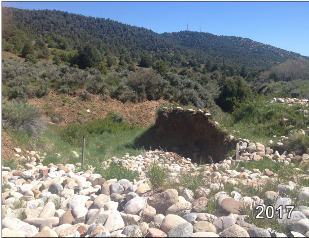
PL-10. (a) Northeast Outflow Channel Bottom Is Stable, Whereas Upland Area on Right Is Slowly Eroding, 2017
