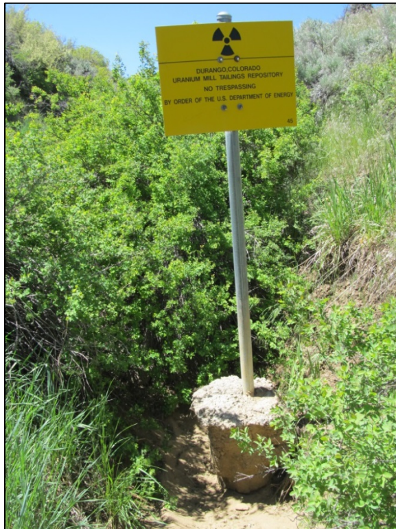
PL-4. Perimeter Sign P45 in Drainage, Entire Base Nearly Standing Free
