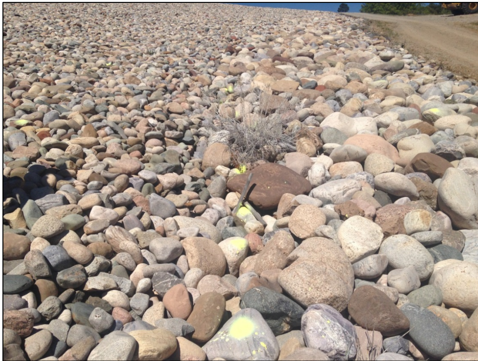
PL-7. View Uphill of 18-Foot Linear Depression on Toe of Northeast Disposal Cell Side Slope (Yellow Paint Marks Centerline of the Depression)
