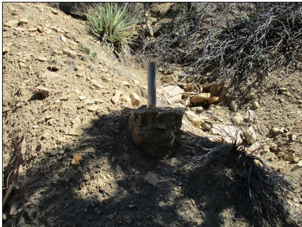
PL-6. Erosion of North Witness Corner of Boundary Monument BM-3 (Addressed Following Inspection)
