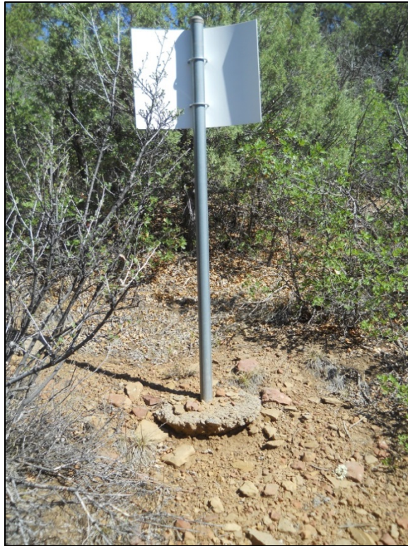
PL-1. Base of Perimeter Sign P62 (Undercut)
