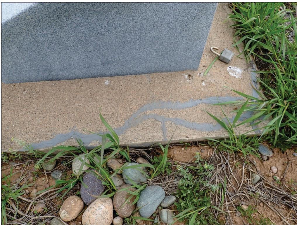
PL-3. 2018 Repairs to Base of Site Marker SMK-2
