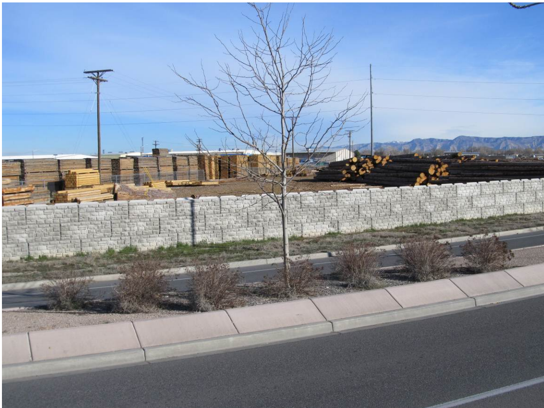
GJT 3/2011. PL-4. Lumber mill storage area and concrete fence within the institutional control boundary.
