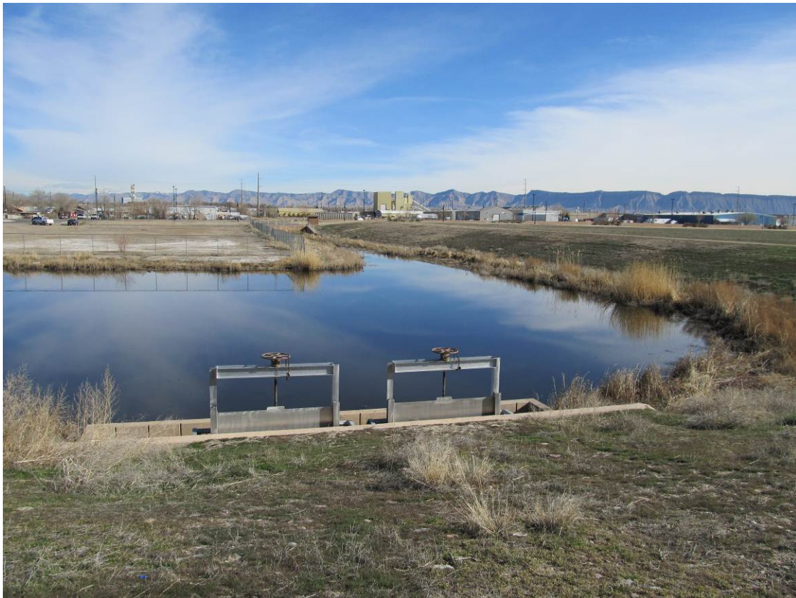
GJT 3/2011. PL-3. Storm water retention basin on the west side of the institutional control area.
