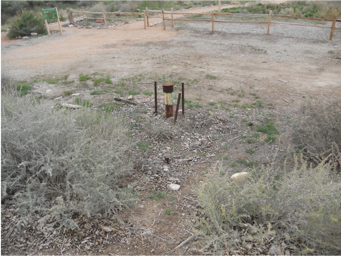
GJT 4/2016. PL-6. Monitoring well MW-0590 with a bent bollard.
