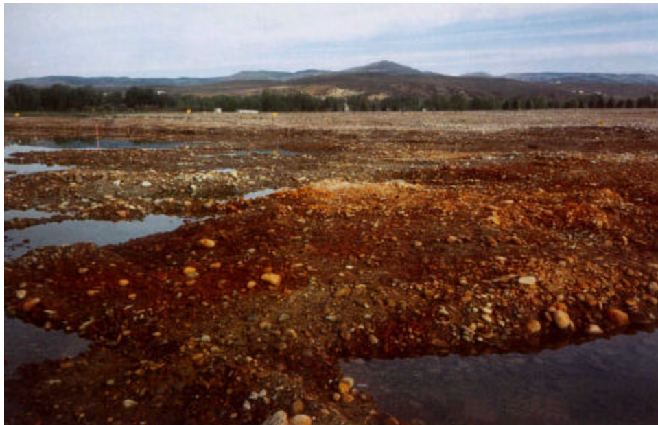
Figure 4–3. Excavated Millsite During Surface Remediation (1994?) (View 2)
