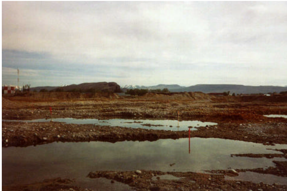
Figure 4–2. Excavated Millsite During Surface Remediation (1994?) (View 1)
