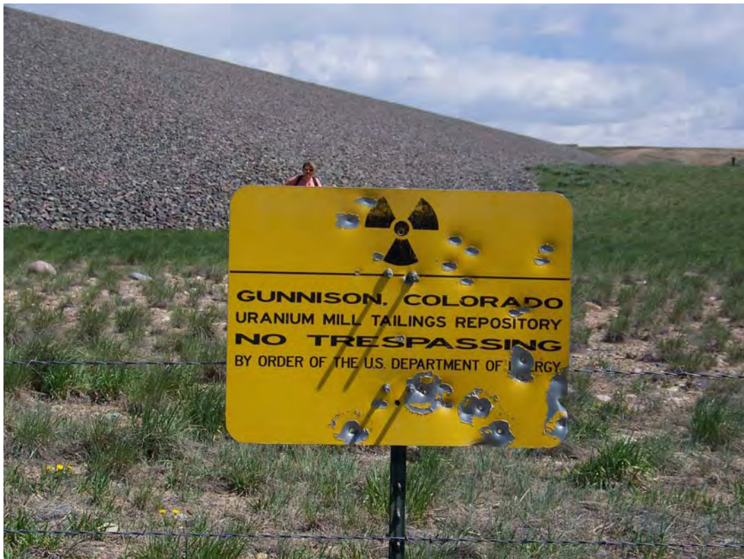
GUN 6/2008. PL-2. Damaged perimeter sign P42.
