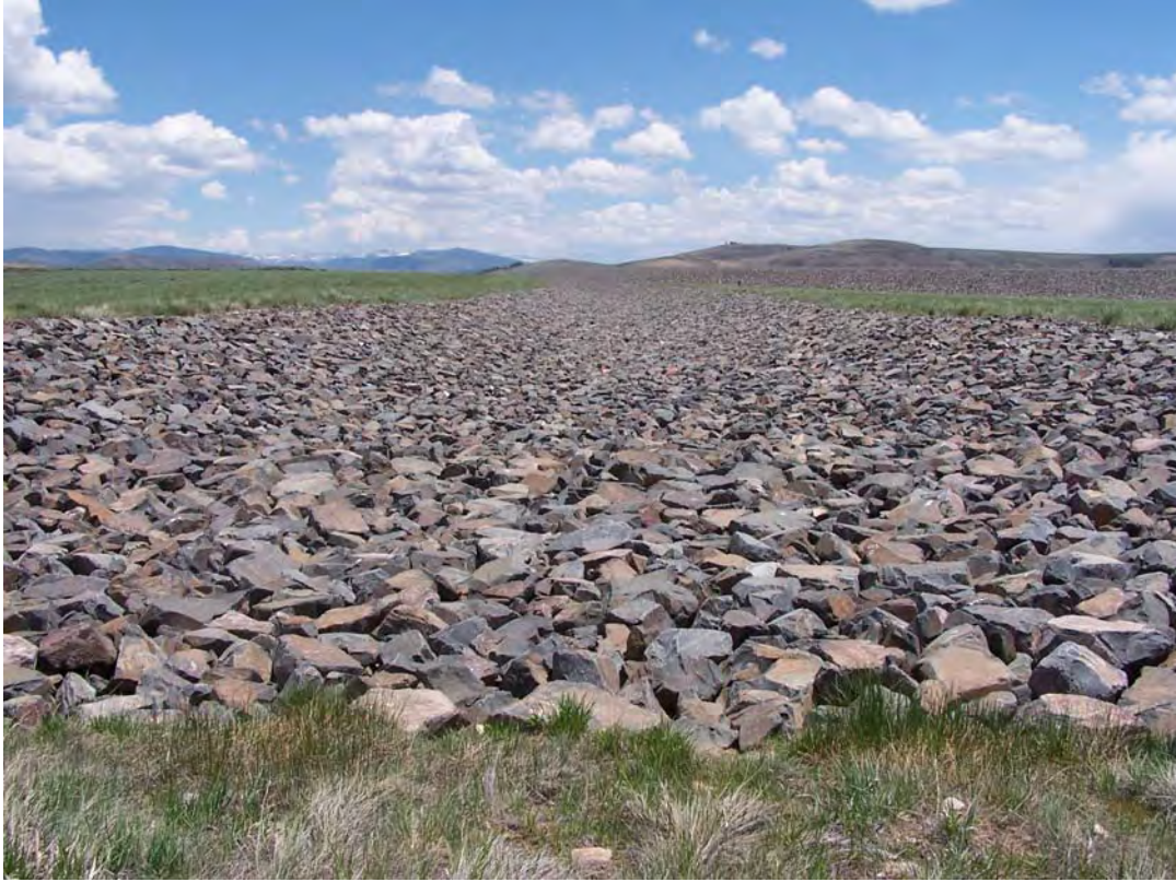
GUN 6/2008. PL-5. West diversion channel.
