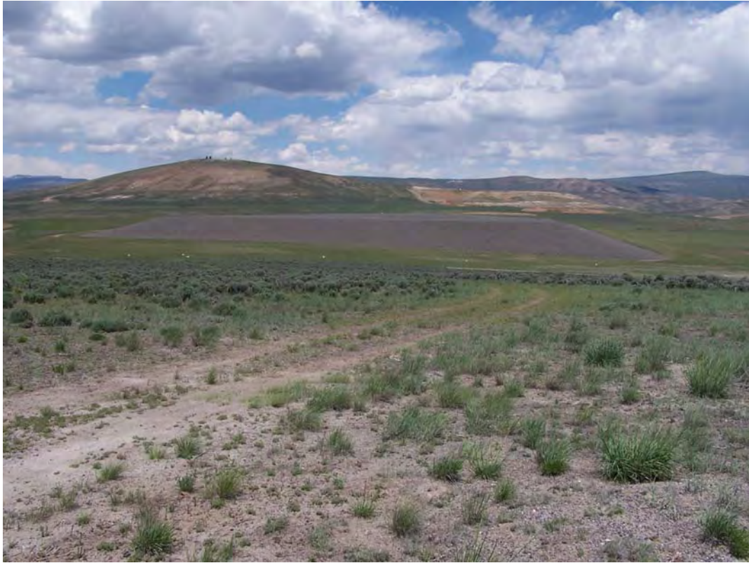
GUN 6/2008. PL-3. Disposal cell viewed from the south.
