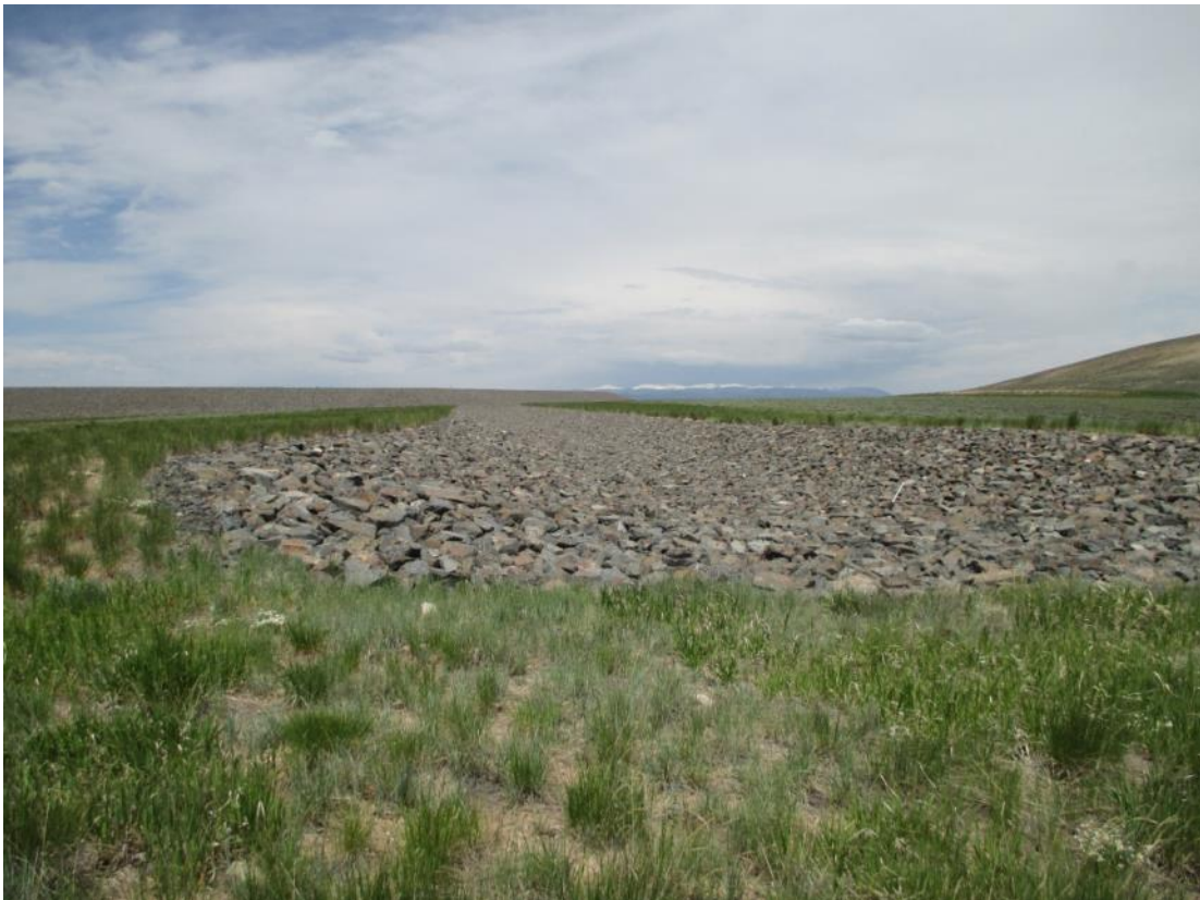
GUD 6/2014. PL-8. East diversion channel.
