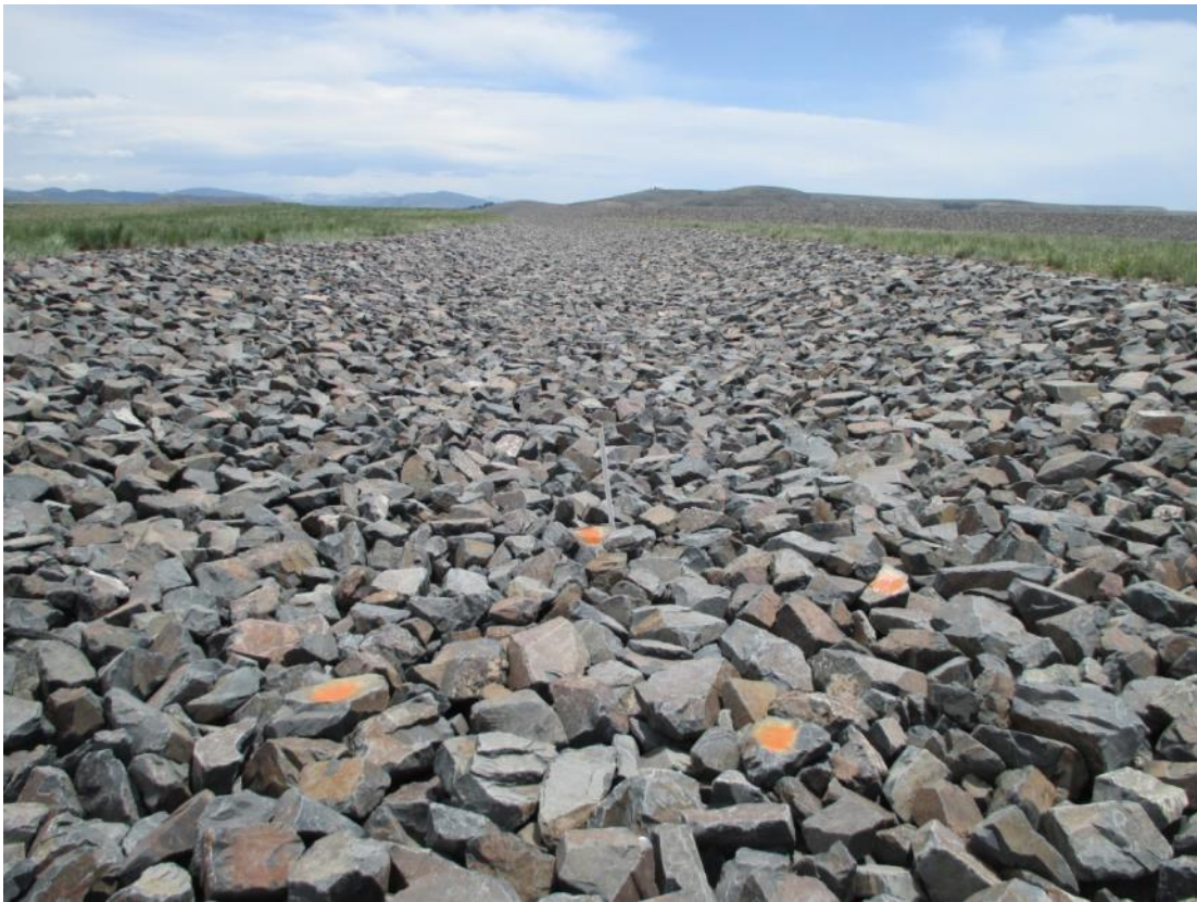
GUD 6/2014. PL-9. West diversion channel; Riprap Test Area No. 6 in foreground.
