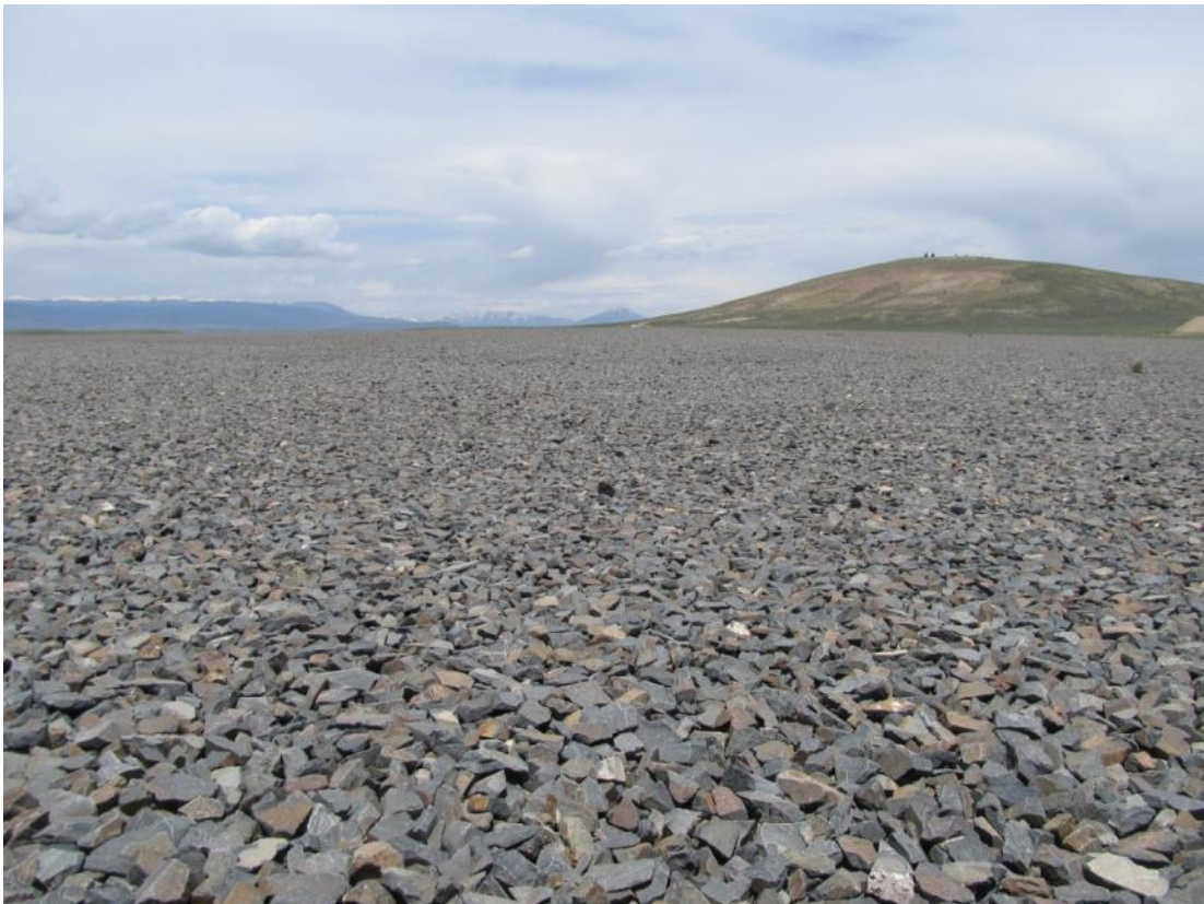
GUD 6/2014. PL-6. Top slope of disposal cell.
