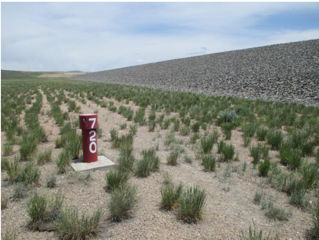
GUD 6/2014. PL-4. Monitoring well 0720 near west side of disposal cell.
