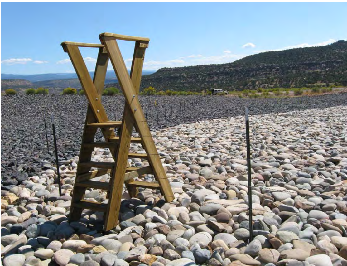
NAD 8/2008. PL-4. New pedestrian fence ladder installed near boundary monument BM-16.
