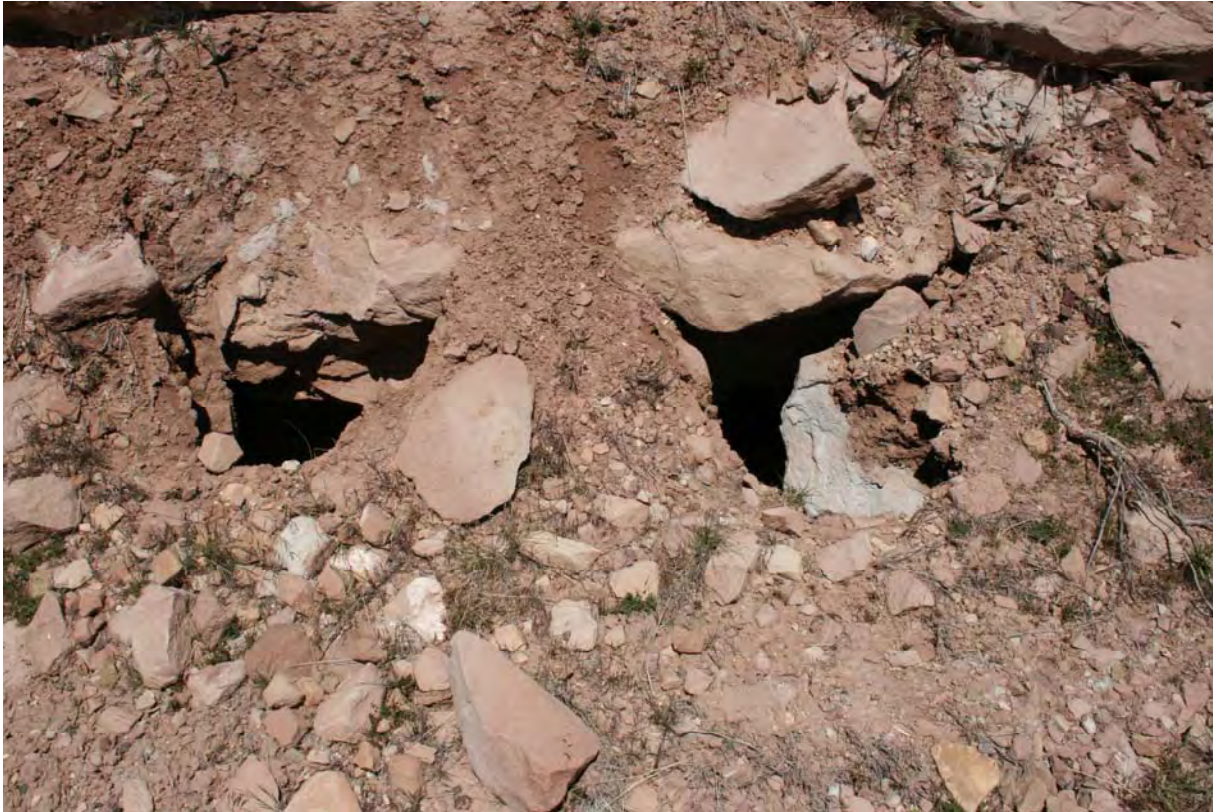
NAD 5/2008. PL-1. Hole eroded along west side of access road near top of hill that leads into cell.
