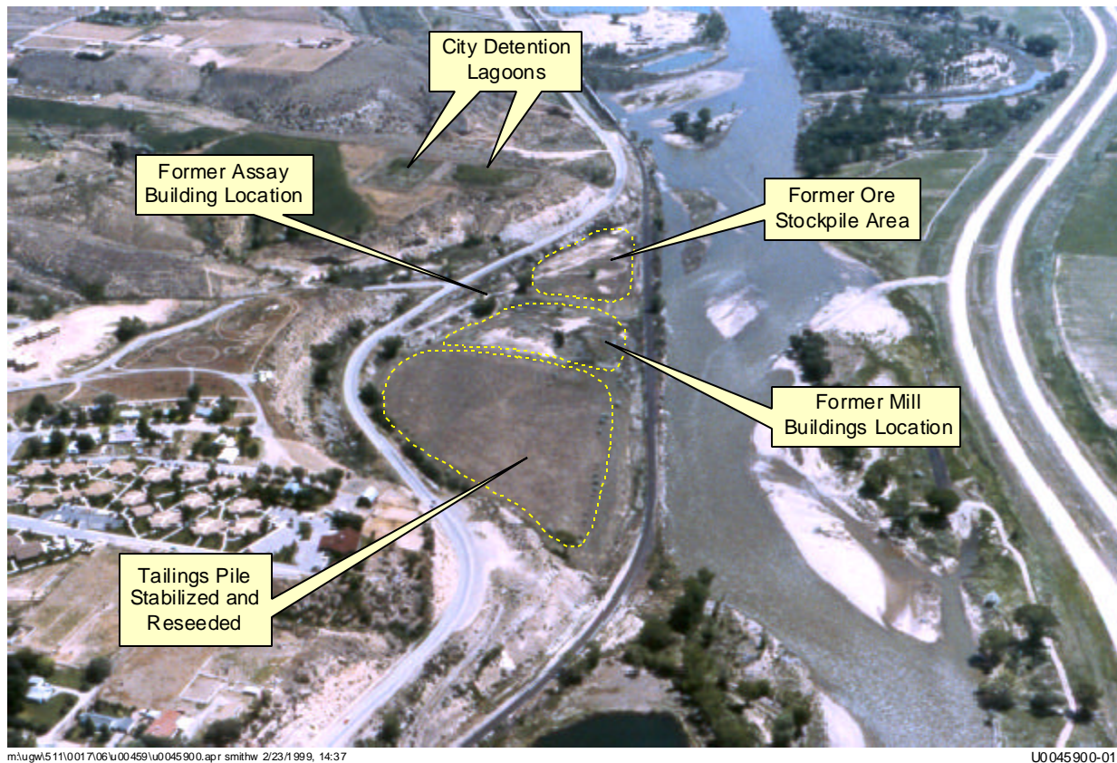
Figure 3-1. Former Tailings Pile, Ore Storage Area, and Associated Buildings at the Old Rifle Site
