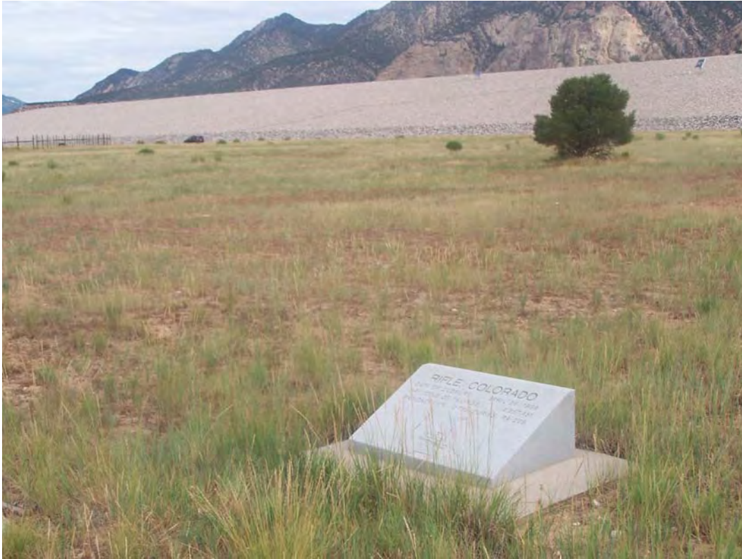
RFL 8/2008. PL-1. Site marker SMK-1 and the south slope of the disposal cell.
