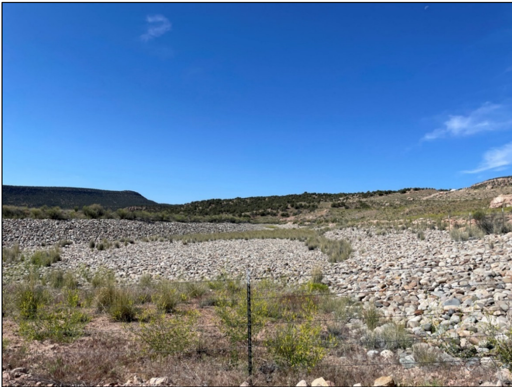
PL-6. Interceptor Trench on North Side of Site
