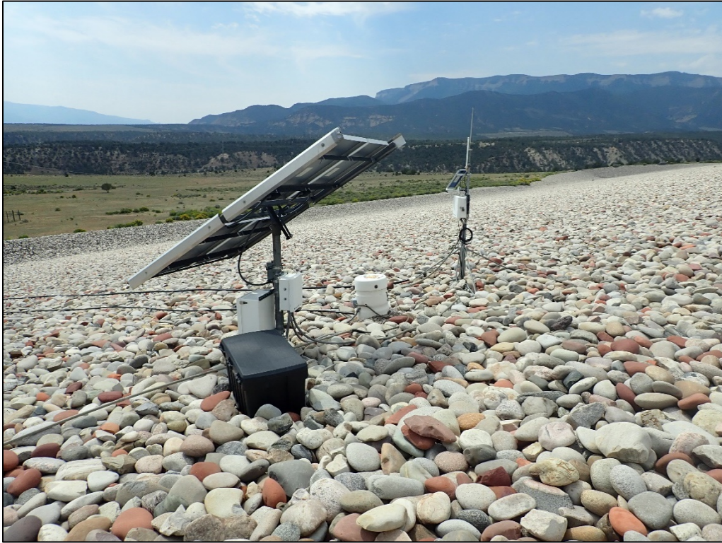
PL-5. Standpipe SP-02 and Instrumentation
