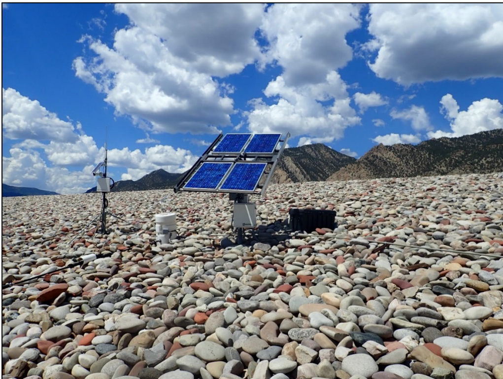
PL-6. Standpipe SP-02 and Instrumentation
