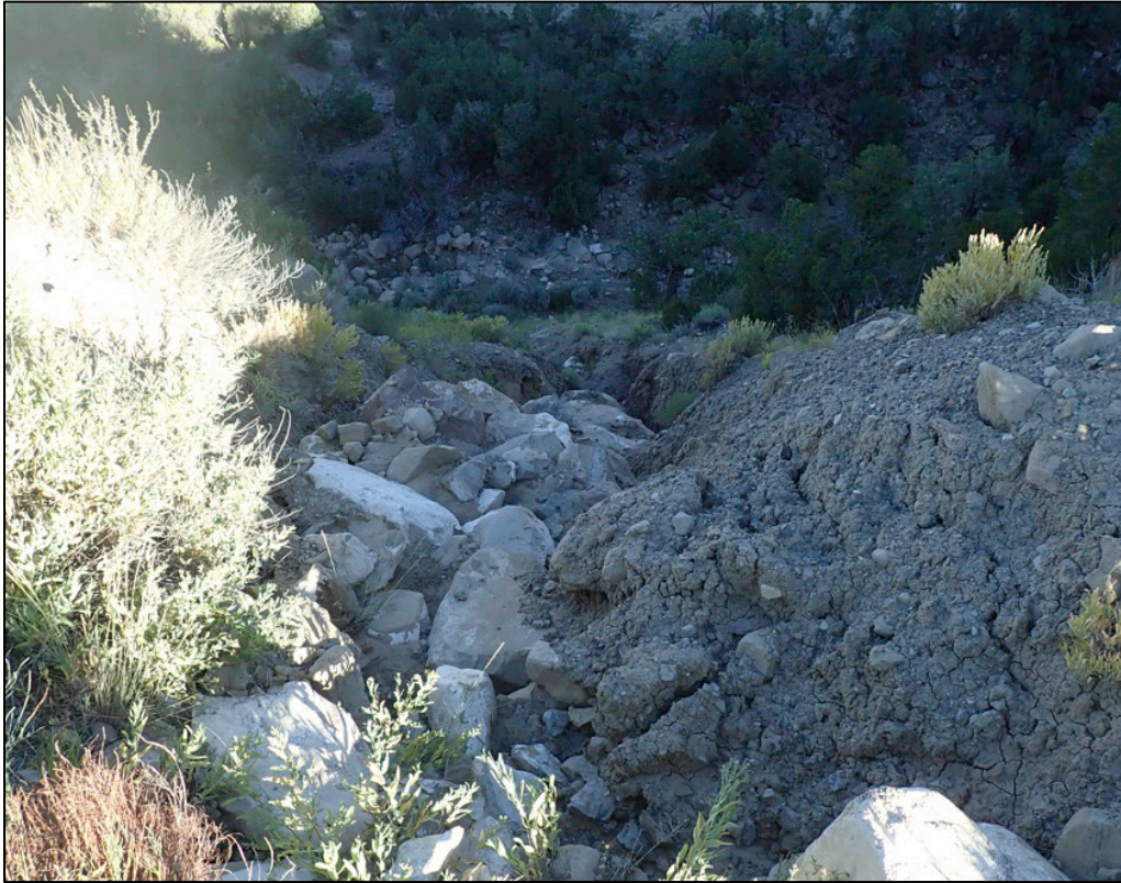
PL-9. Gully at Toe of Interceptor Trench
