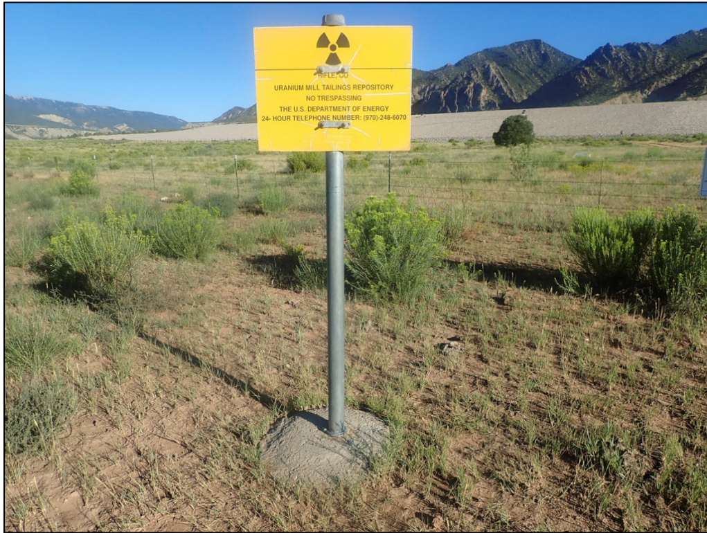
PL-1. Entrance Sign, Cracked and Faded but Legible
