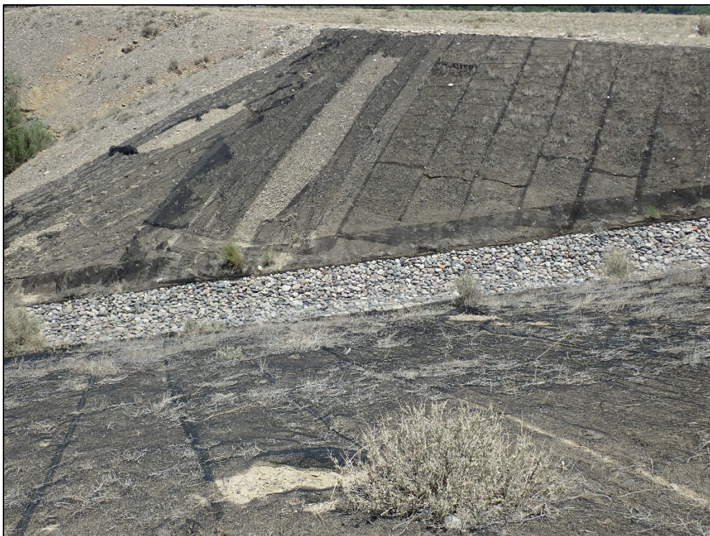
PL-10. Torn Areas in Erosion Control Fabric on Northwest End of Outflow Channel
