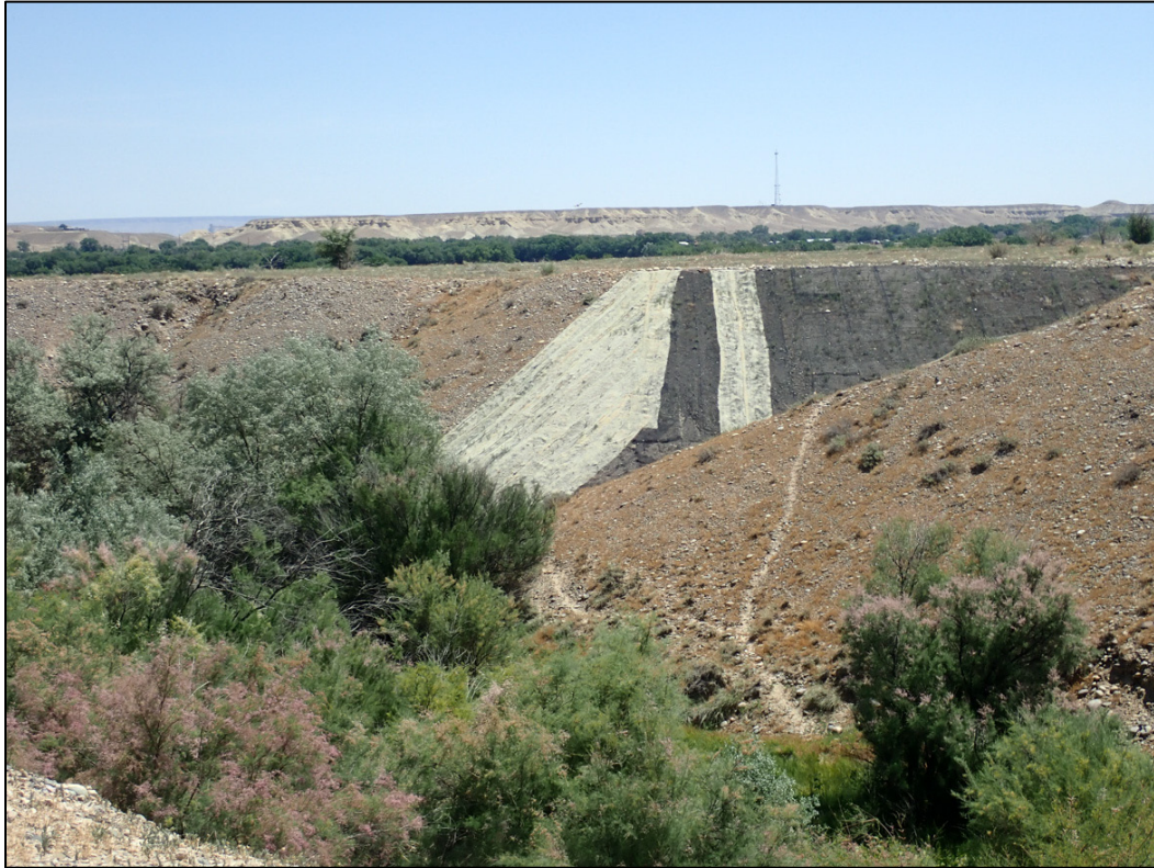
PL-7. Repaired Erosion Control Fabric
