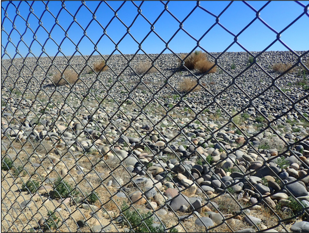
PL-5. Treated Vegetation on Side Slope
