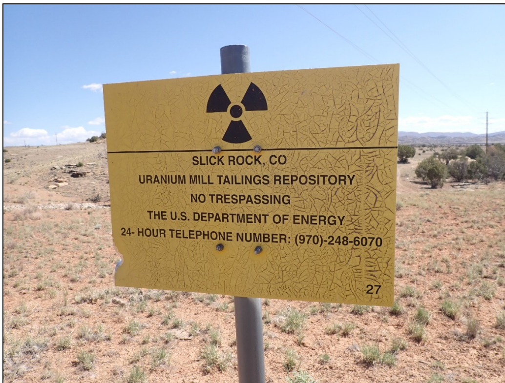
PL-2. Cracked Overlay on Perimeter Sign P27
