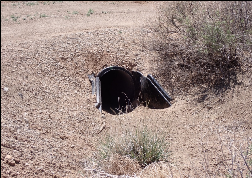
PL-8. North Side of Culvert Under Access Road Inside Gate
