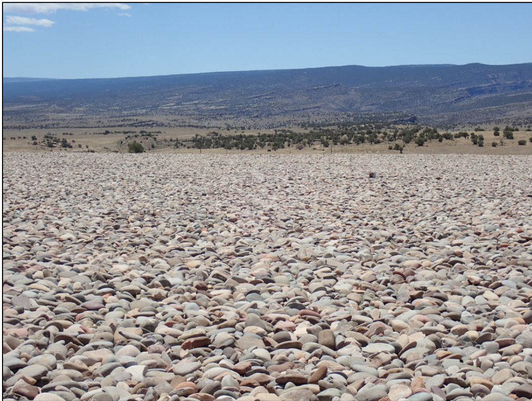
PL-4. Disposal Cell Top Slope
