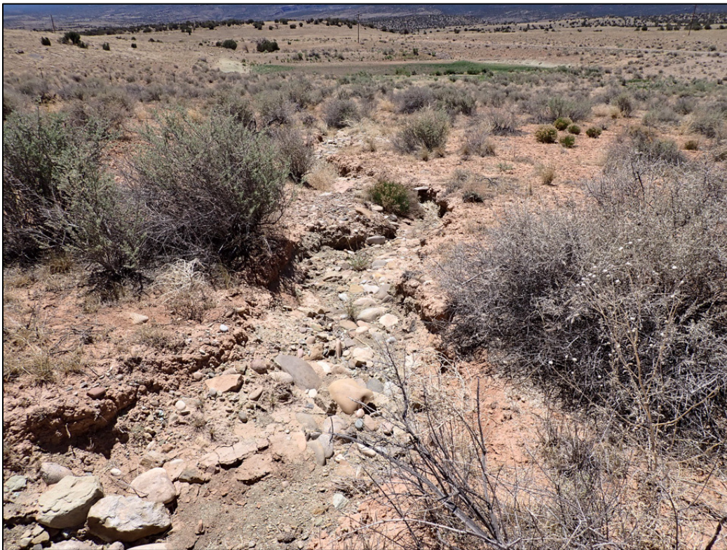
PL-8. Gullies on South Area Between Disposal Cell and Site Boundary
