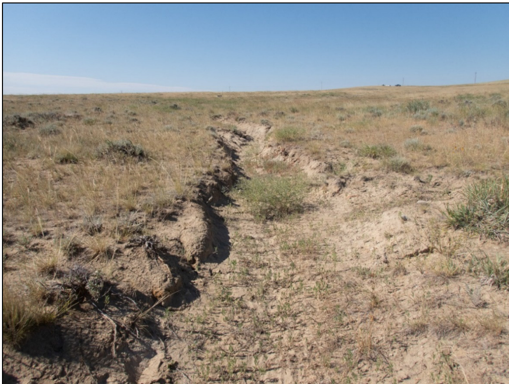
PL-6. Erosional Gully, Previously Unreported
