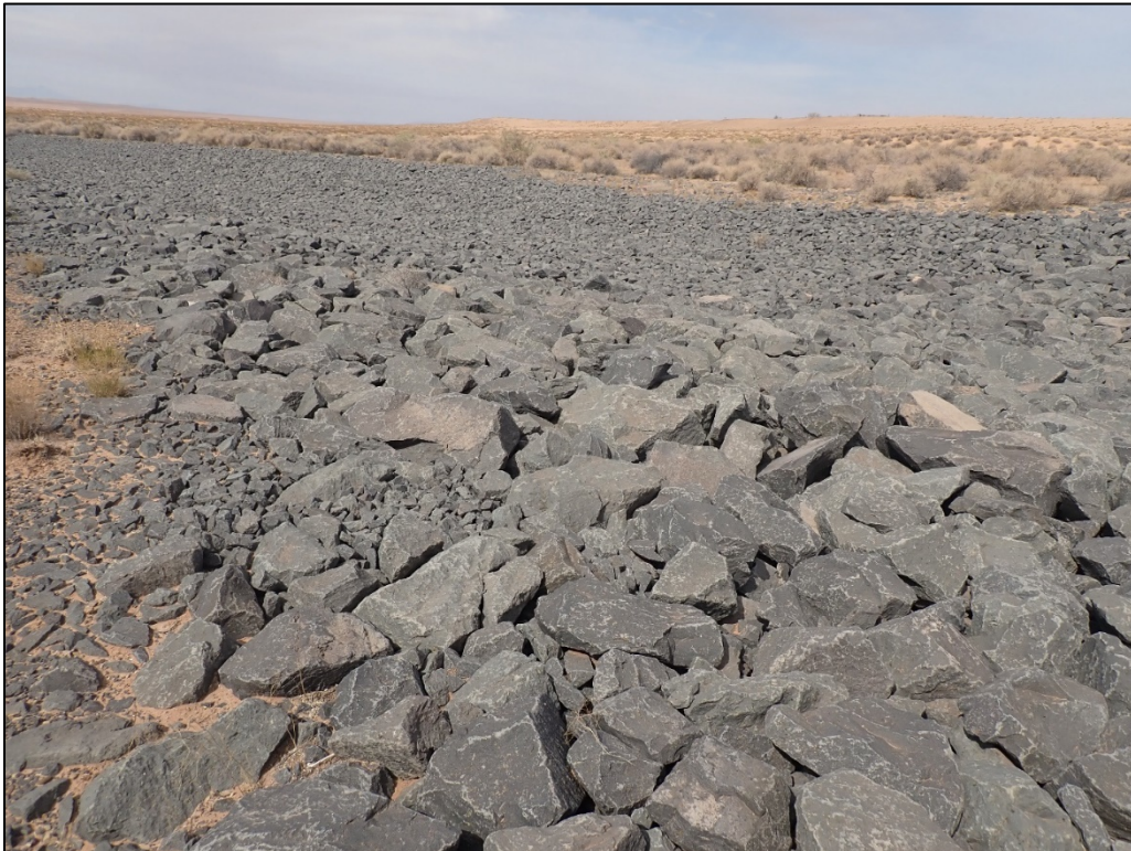
PL-10. Minor Sedimentation and Plant Growth in Mouth of South Apron Ditch
