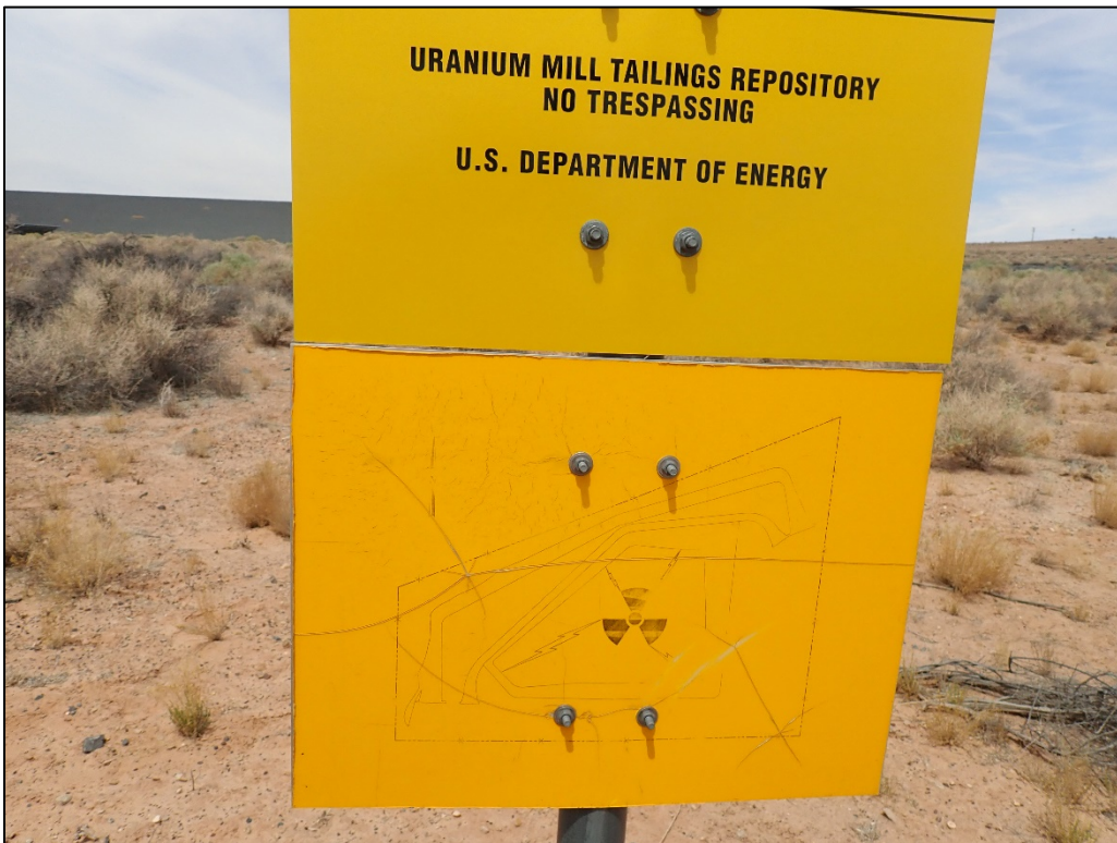
PL-4. Faded and Cracked Pictorial Perimeter Sign P24
