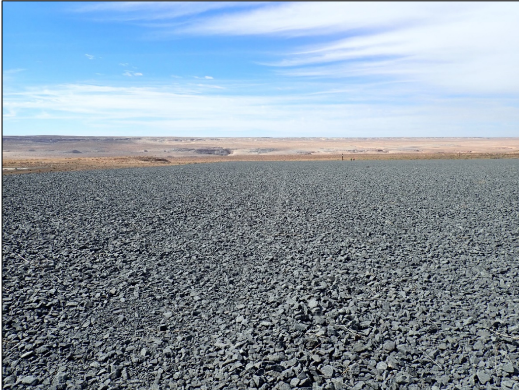
PL-9. Tire Tracks on Disposal Cell Top
