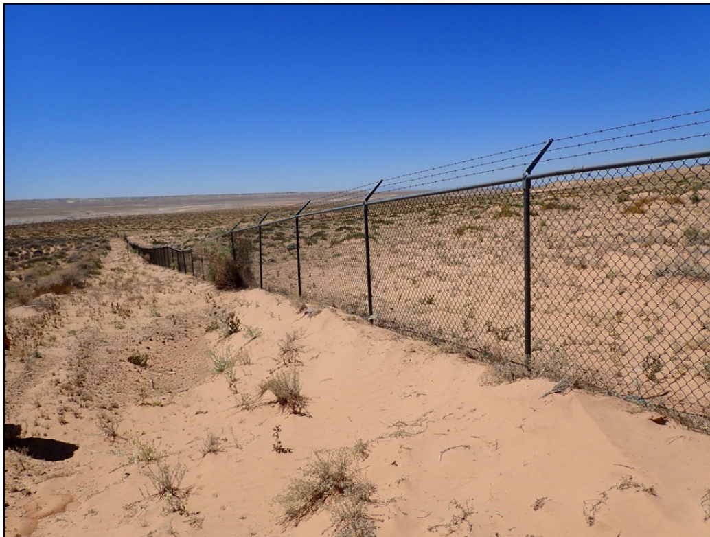
PL-2. West Perimeter Fence with Sand Deposition
