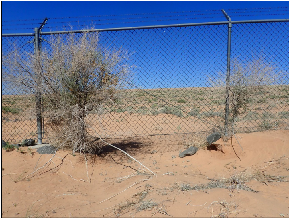
PL-1. Gap Under Fence near Perimeter Sign P9
