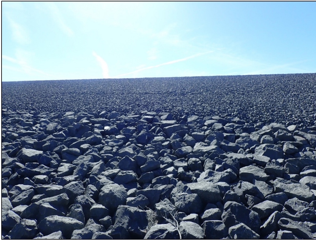
PL-9. Horizontal Lines on West Slope of Disposal Cell
