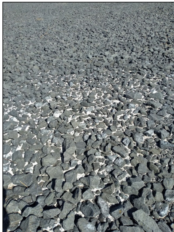
PL-8. Evaporative Minerals on Top Slope of Disposal Cell
