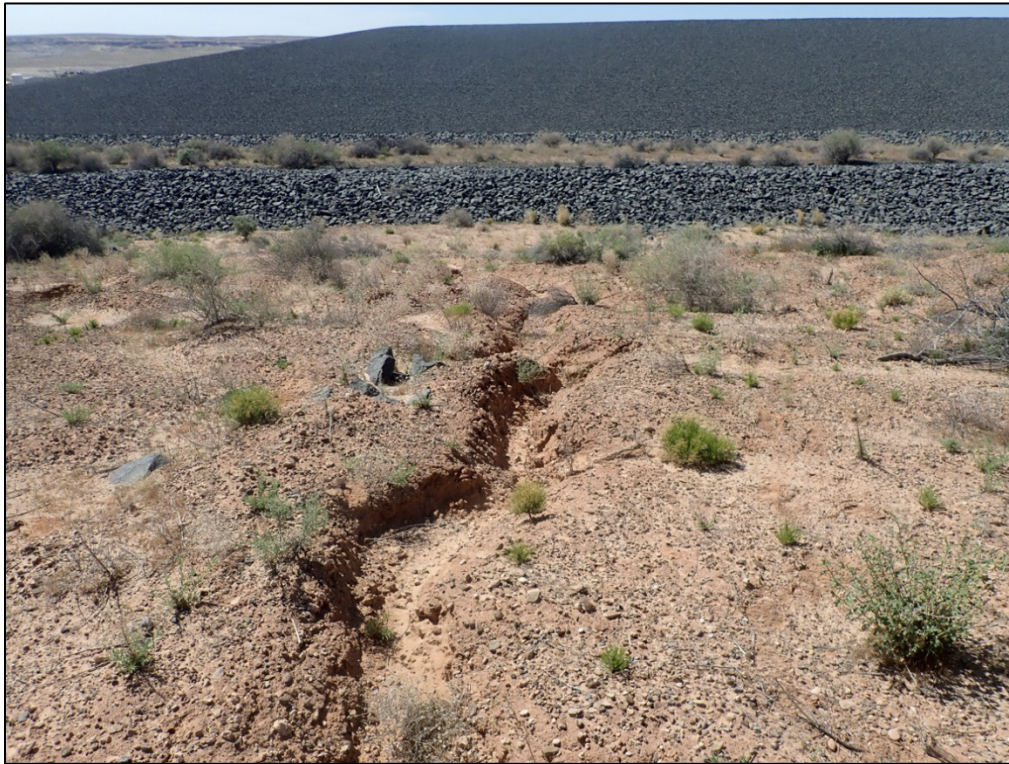
PL-11. Erosion Gully and Soil Accumulation in Diversion Ditch North of Disposal Cell
