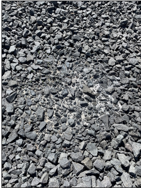
PL-7. Evaporative Materials on Top Slope of Disposal Cell
