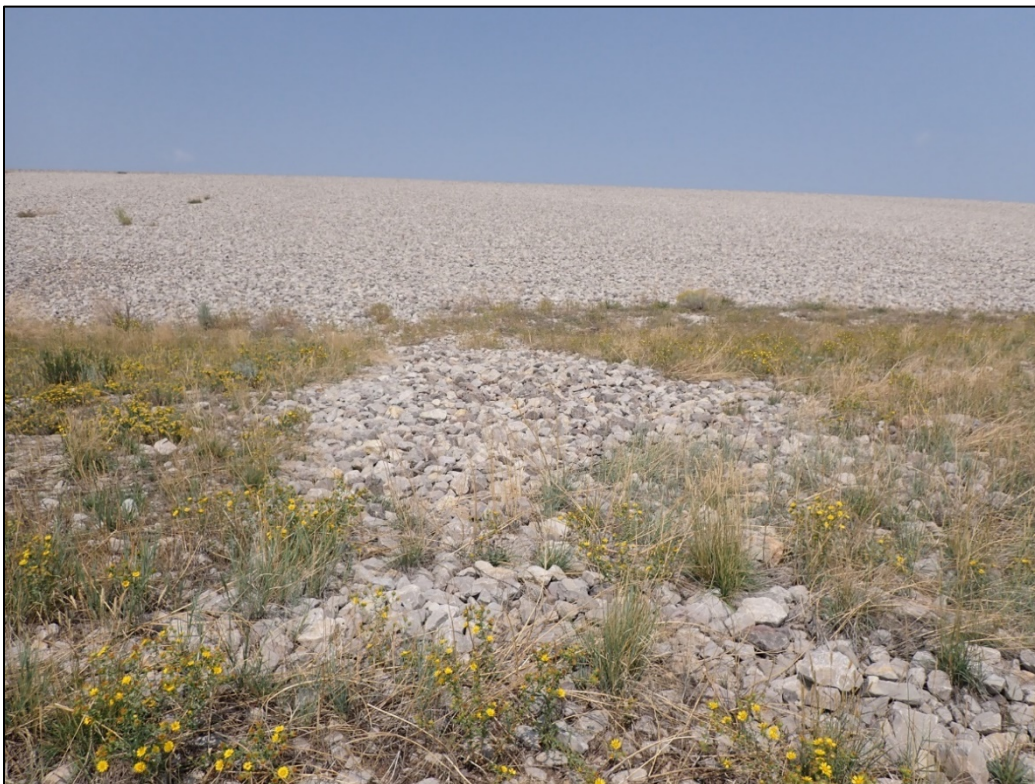
PL-12. Apron Toe Drain on the South Side of Disposal Cell
