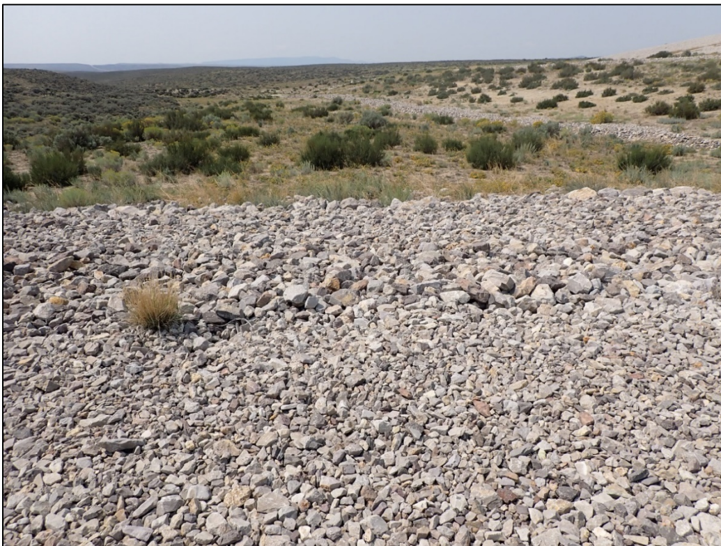
PL-14. Small Depressions on Ancillary Cell Top Slope
