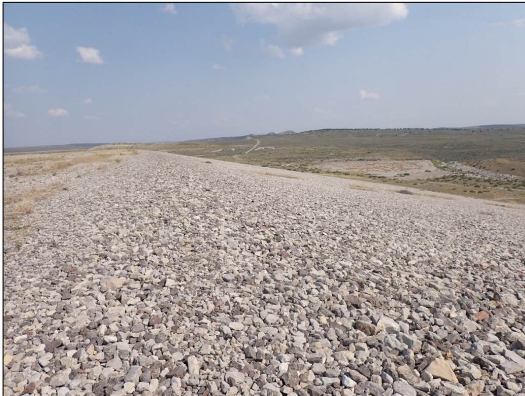
PL-10. View Southeast of Southern Disposal Cell Side Slope
