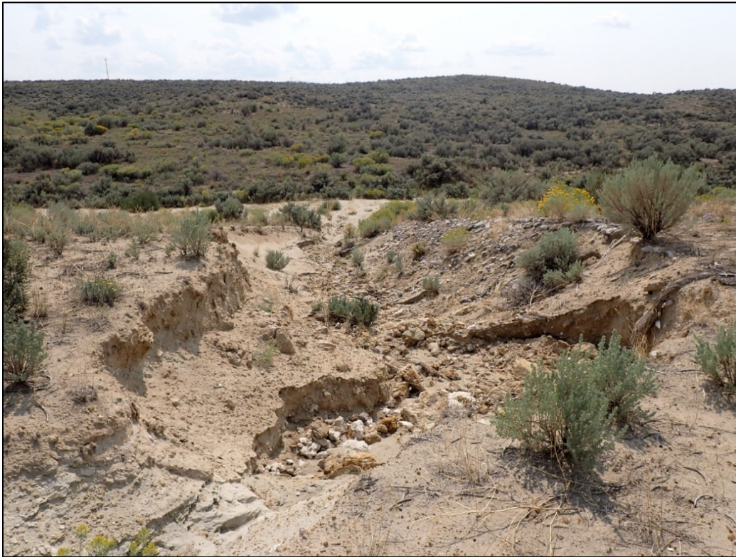
PL-17. Erosion South of Rock Berm Near Diversion Channel No. 2
