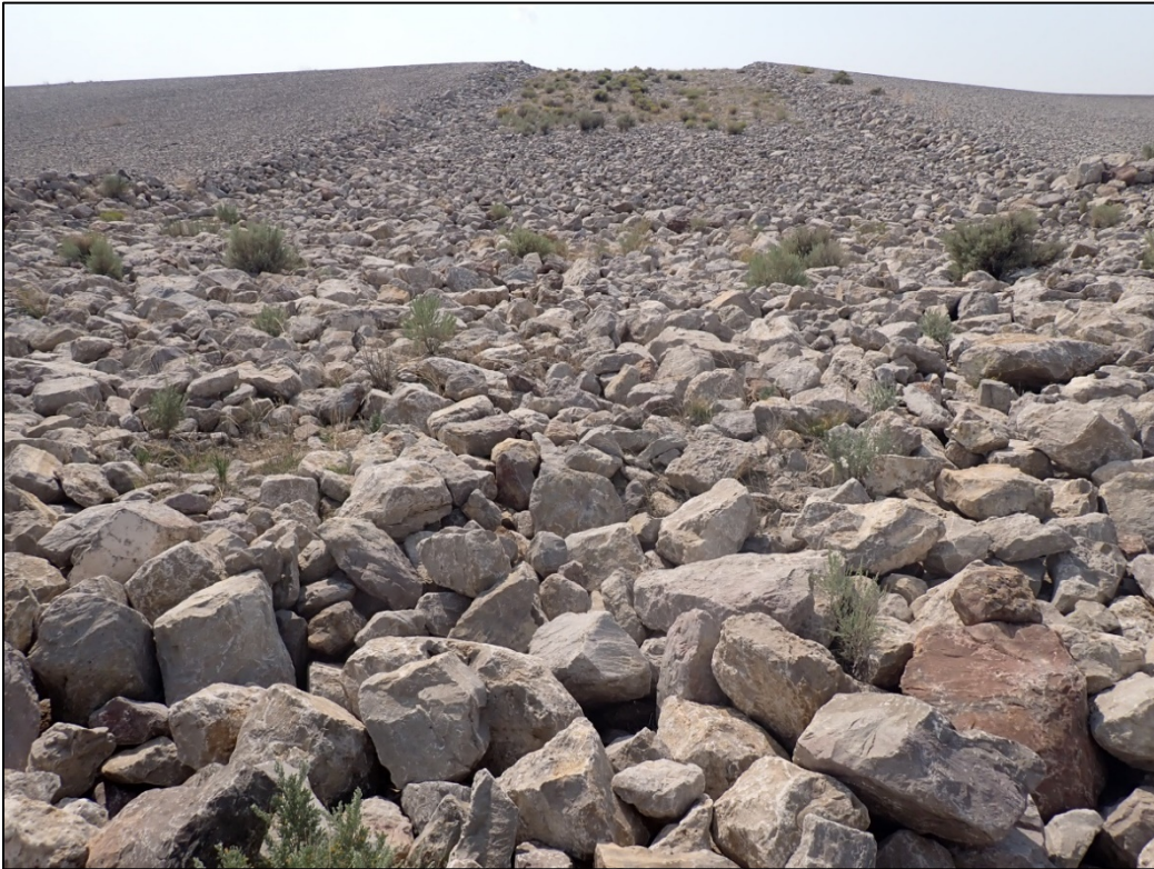
PL-16. View Southwest of the Launch Rock Erosion Protection Basin
