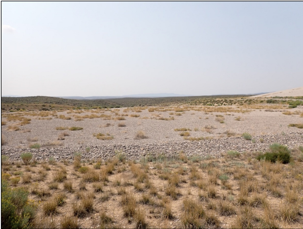
PL-13. View West of Ancillary Cell Top Slope
