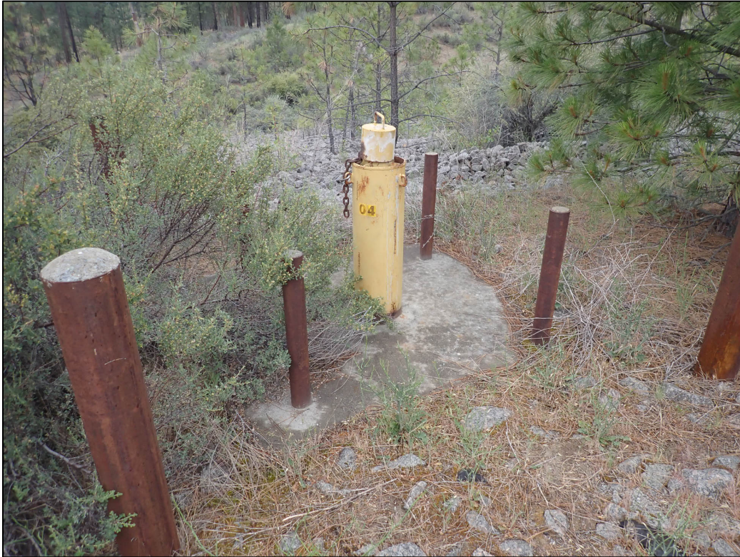
PL-5. Monitoring Well 4
