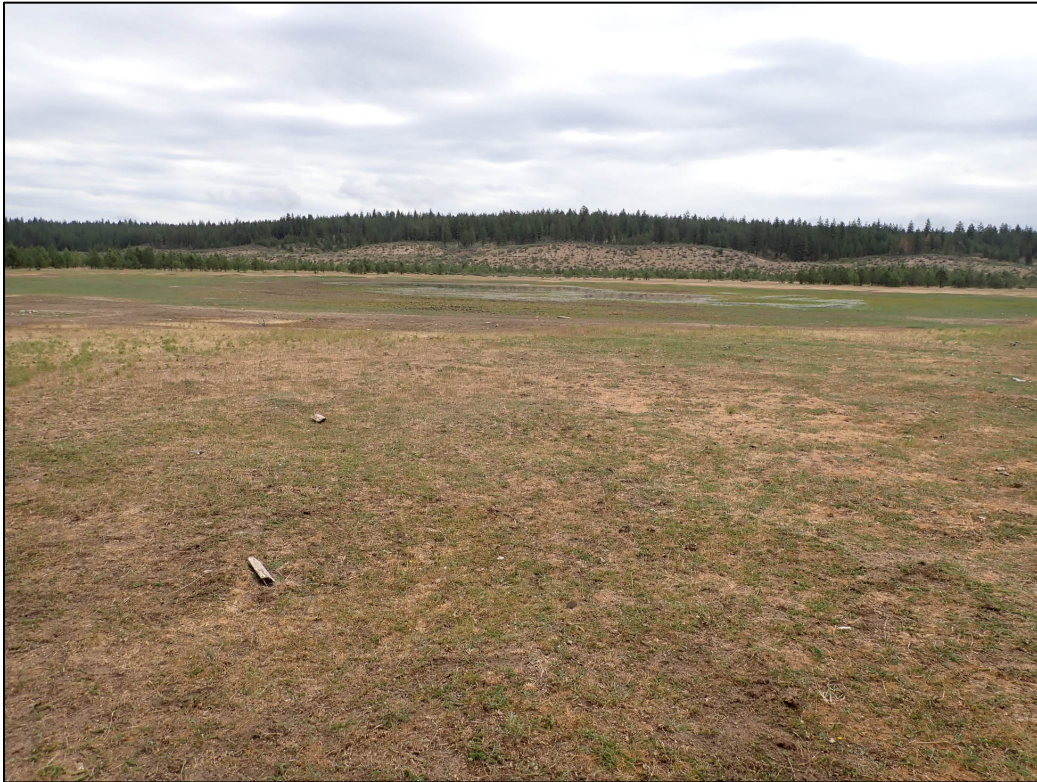
PL-10. Disposal Cell Pond 1
