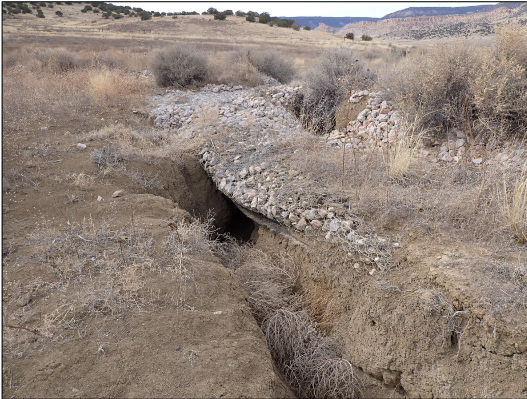
PL-17. Erosion at Structure A
