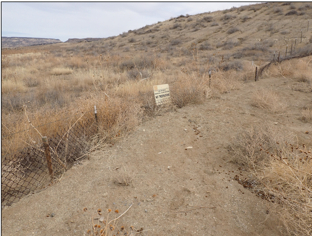
PL-2. Partially Buried Fence from Sedimentation near Perimeter Sign P18
