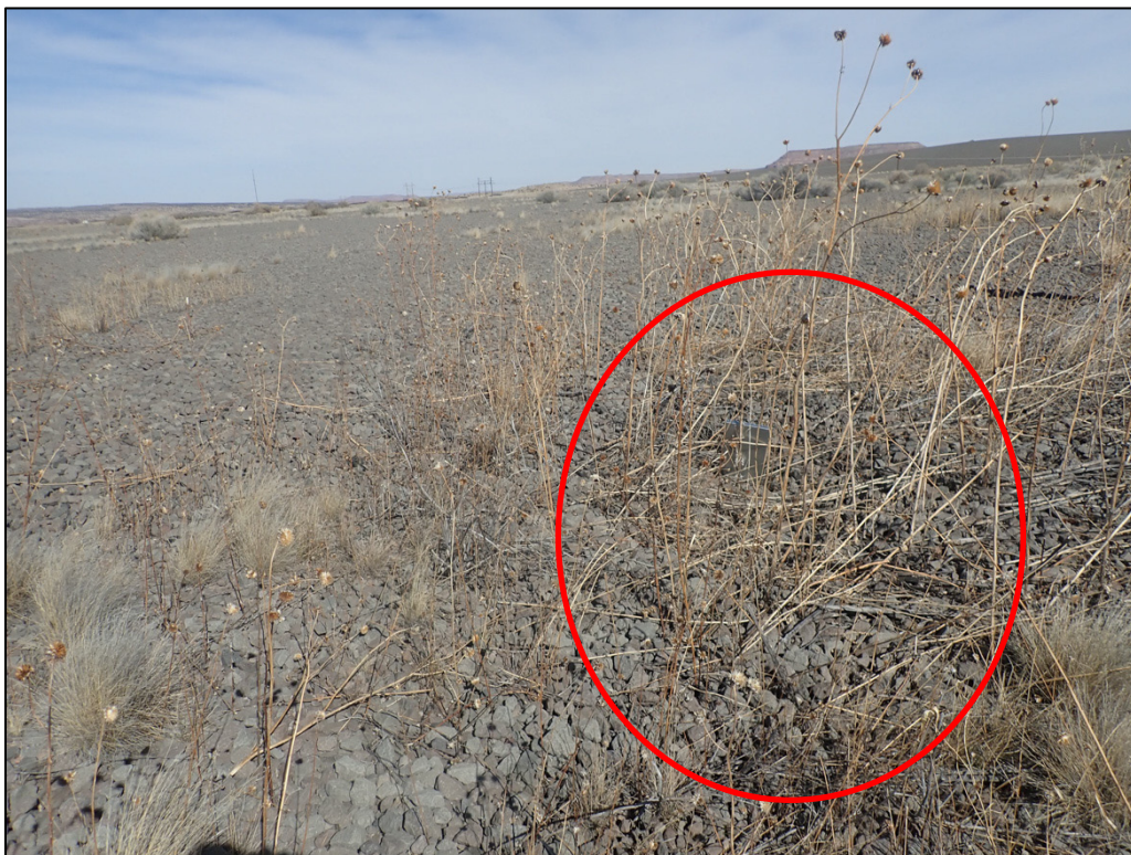
PL-21. Minor Depression with Vegetation Growth on Carbonate Tailings Disposal Cell Top Slope
