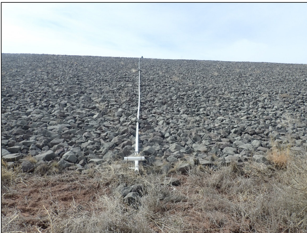
PL-12. Siphon Outlet on Main Tailings Disposal Cell North Side Slope
