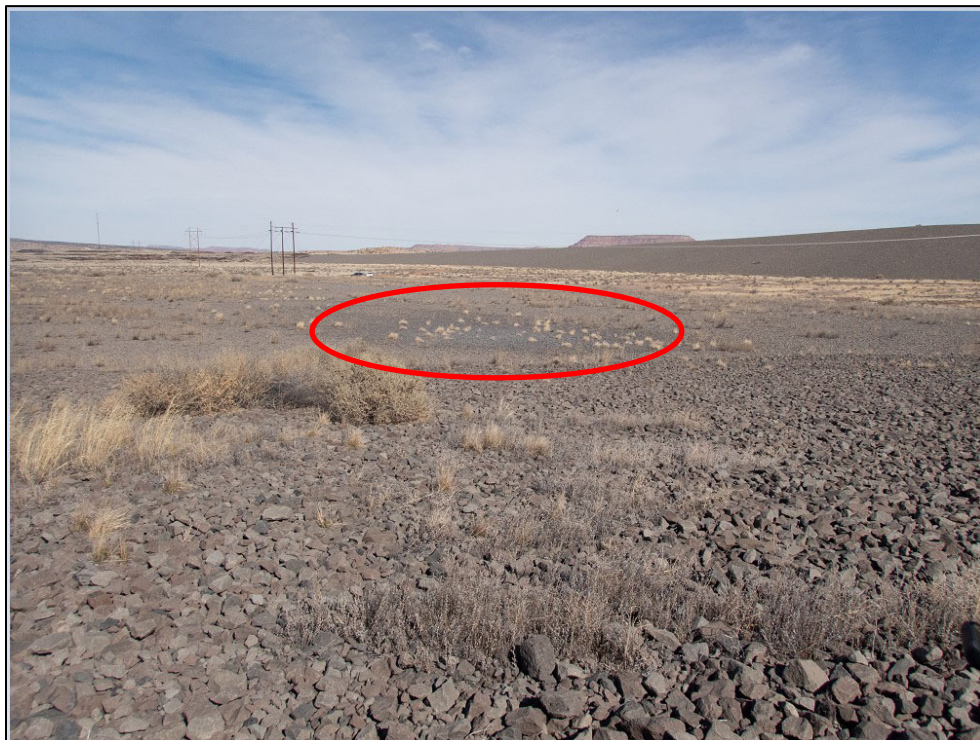
PL-20. Shallow Depression on Northwest Extension of Carbonate Tailings
