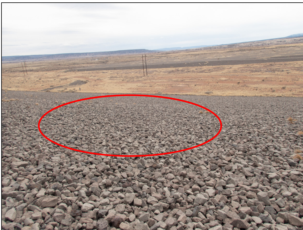
PL-14. Potential Depression Area on Main Tailings Disposal Cell Southwest Side Slope
