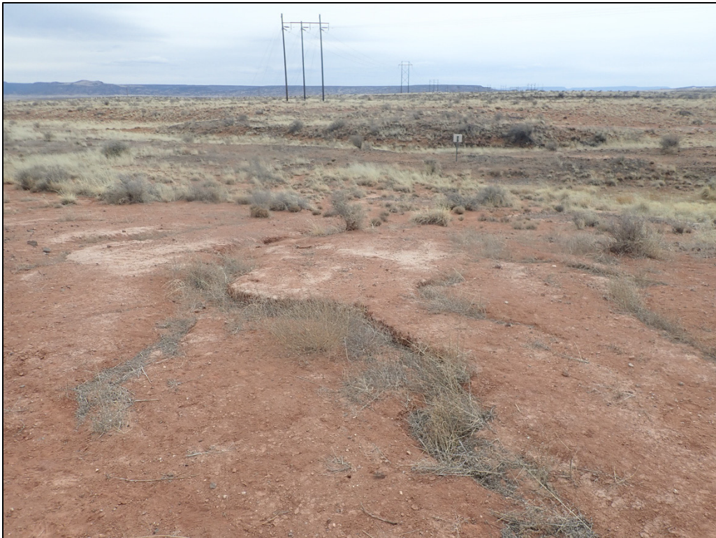
PL-18. Rilling near Perimeter Sign P24
