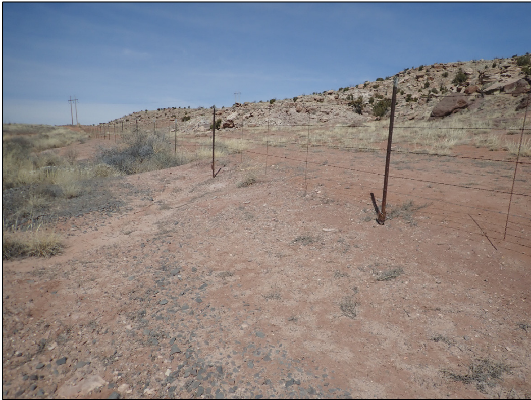
PL-3. Hanging T-Posts Between Boundary Monuments BM-12 and BM-11
