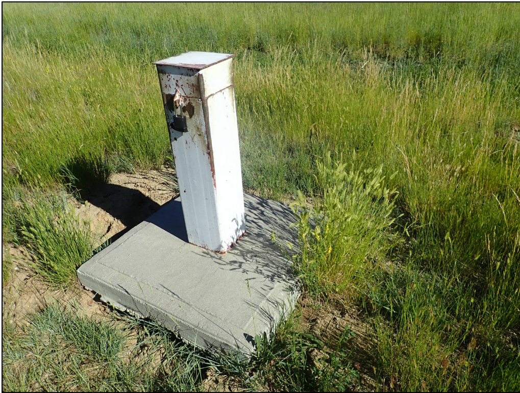
PL-5. Burrowing Near Monitoring Well 40-SC
