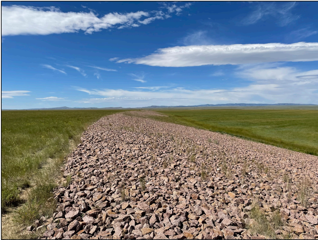
PL-9. Vegetation Encroachment on Upper Riprap Slope
