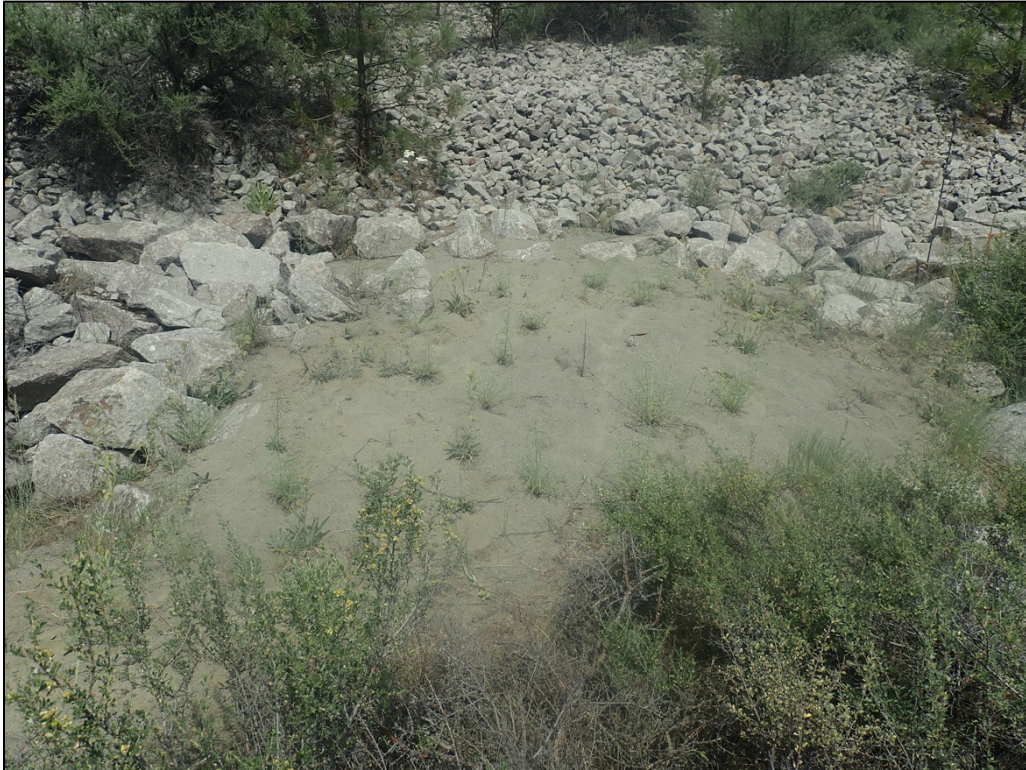
PL-9. Sand Deposit on Containment Dam
