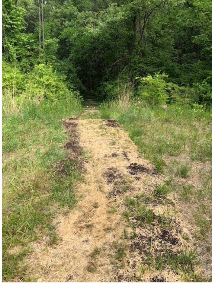
P22 – Erosion Control Application at Plot M
