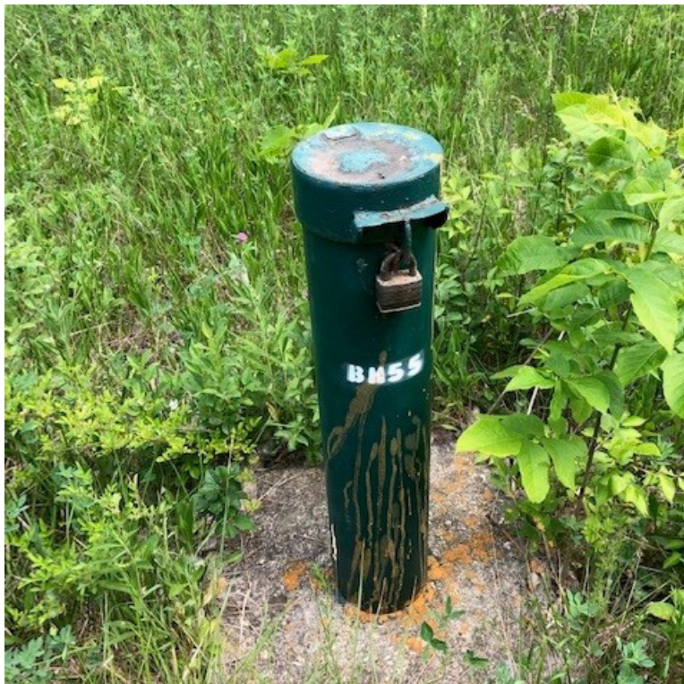
P10 – Monitoring Well BH55 at Site A
