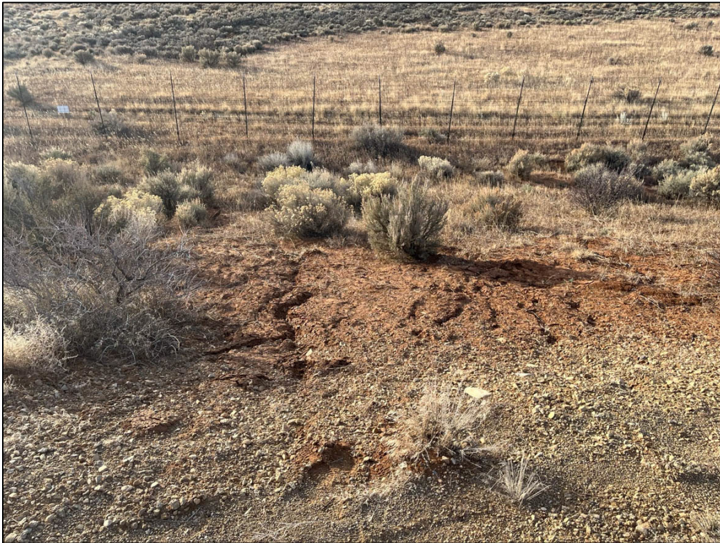
PL-14. Erosion on the South Slope of Pond 4 Berm, Looking South
