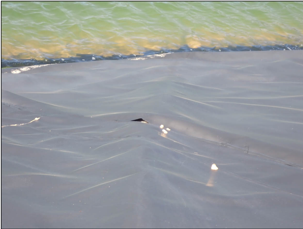
PL-18. Pond 4 Liner Seam Hole on East Side
