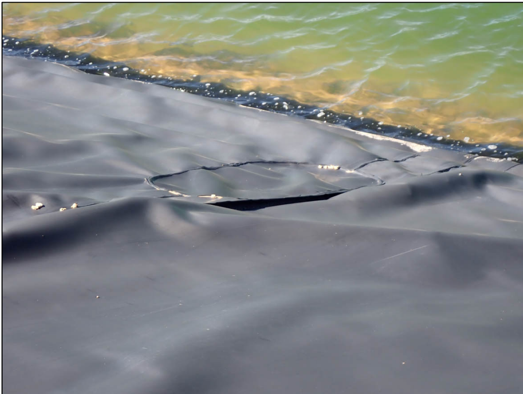
PL-19. Pond 4 Liner Hole on East Side
