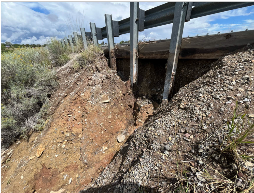
PL-33. Erosion on West Side of Highway 191 Embankment, Looking North
