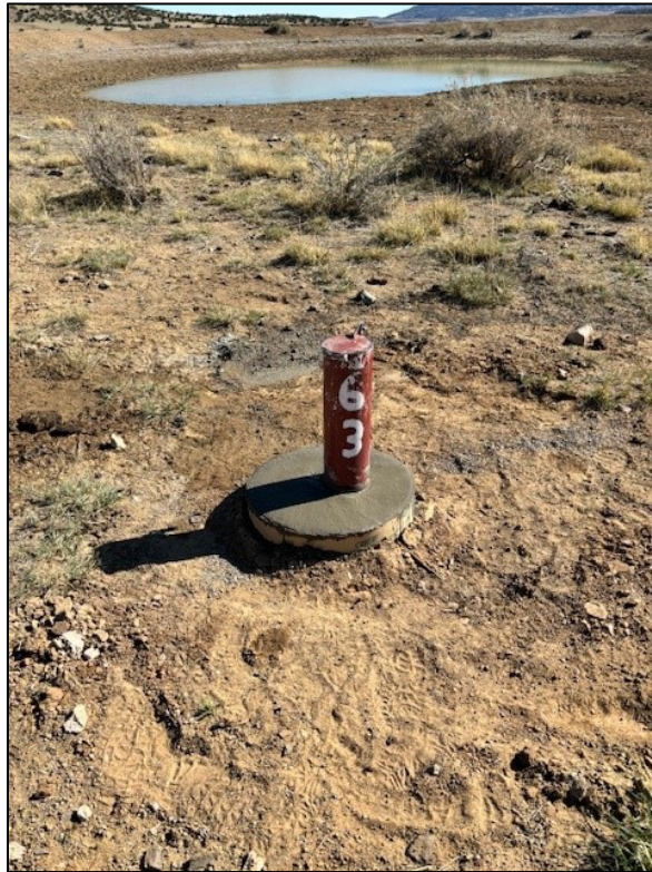
PL-9. New Concrete Pad at Monitoring Well 63
