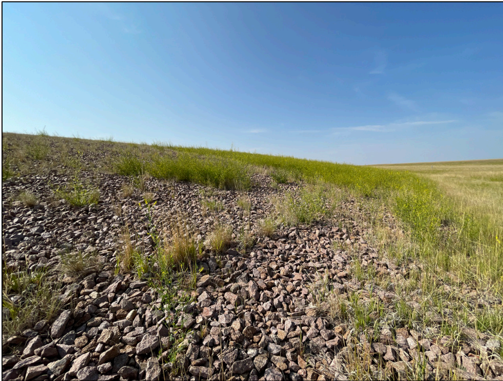
PL-7. Vegetation Encroachment on Lower Riprap Slope
