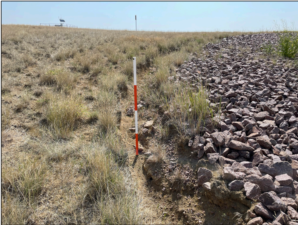
PL-5. Erosion Caused by Animal Trail North of Upper Riprap Slope
