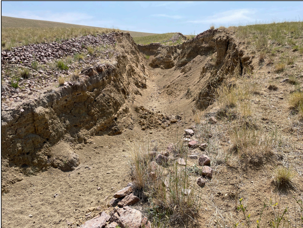
PL-10. Pit 4 Lower Riprap-Armored Drainage Channel Erosion
