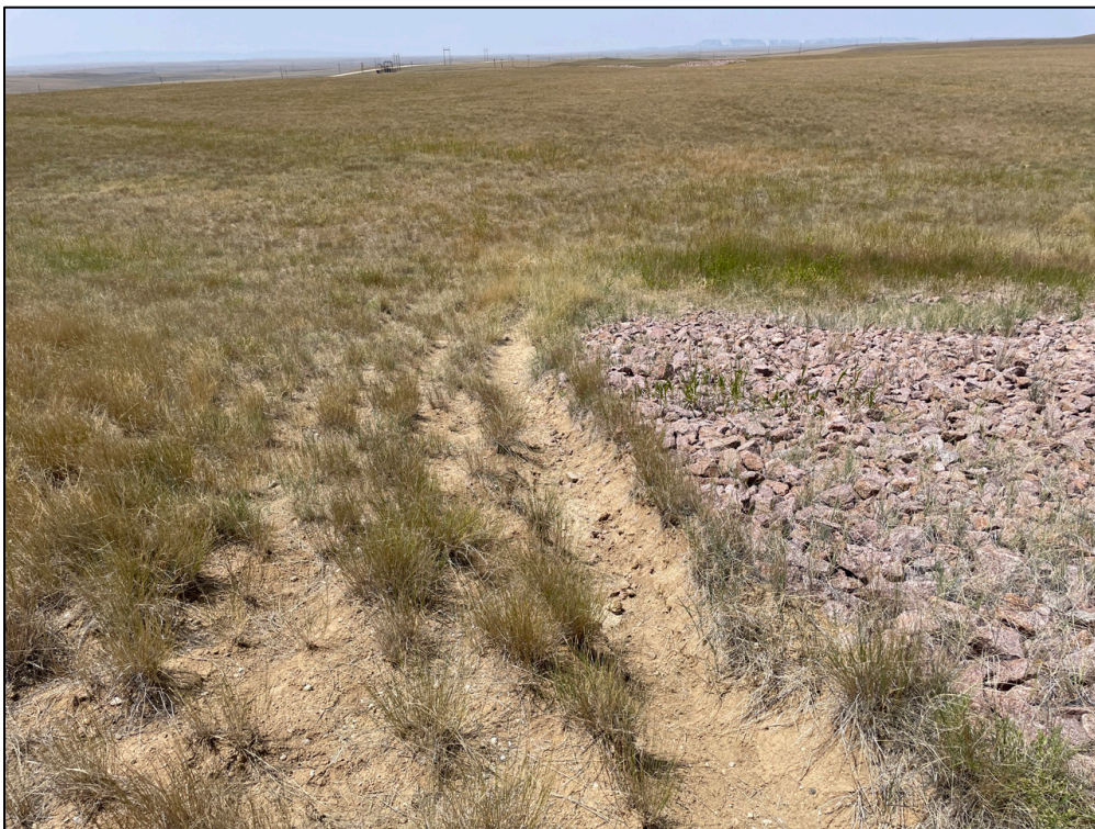
PL-6. Erosion Caused by Animal Trail South of Upper Riprap Slope
