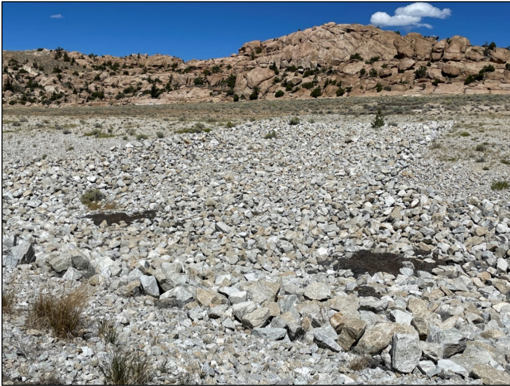
PL-17. Swale Inlet Channel on Disposal Cell
