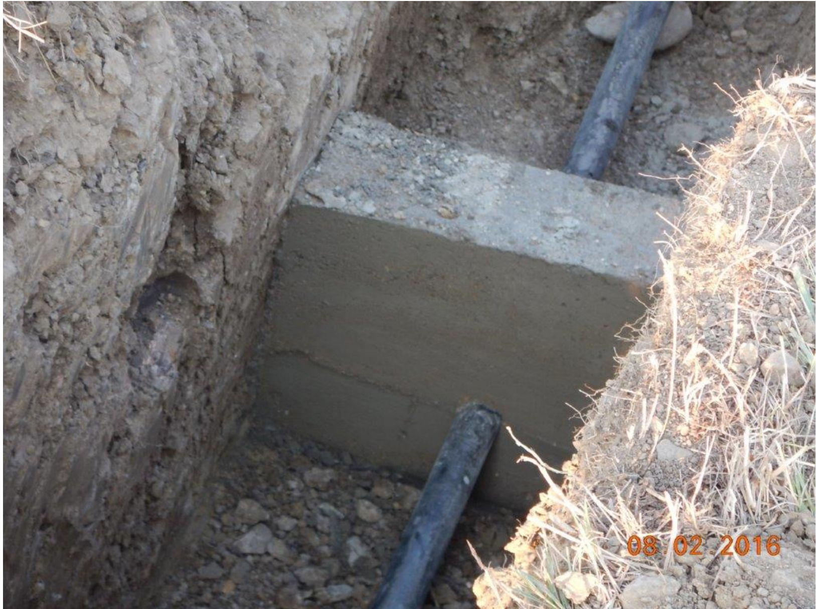
Figure 4. Present Concrete Cut-off Collar at Installation
