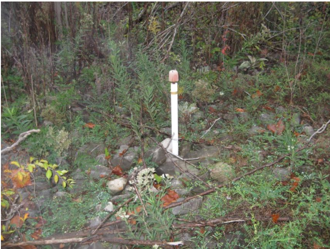
BUR 10/2014. PL-14. Outlet of French drain.
